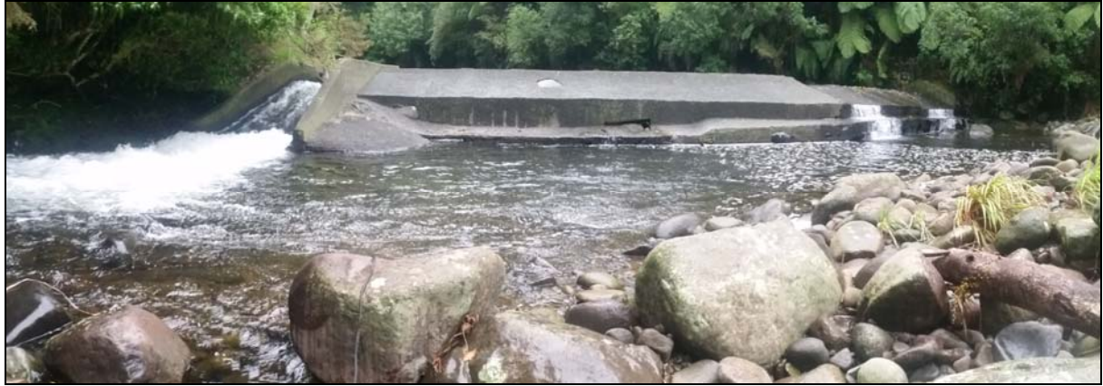
Photo 1 The Scout Road weir, 23 March 2016.
