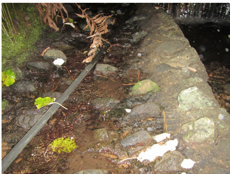
Photo 2 The fish pass with very little flow, 20 April 2016
