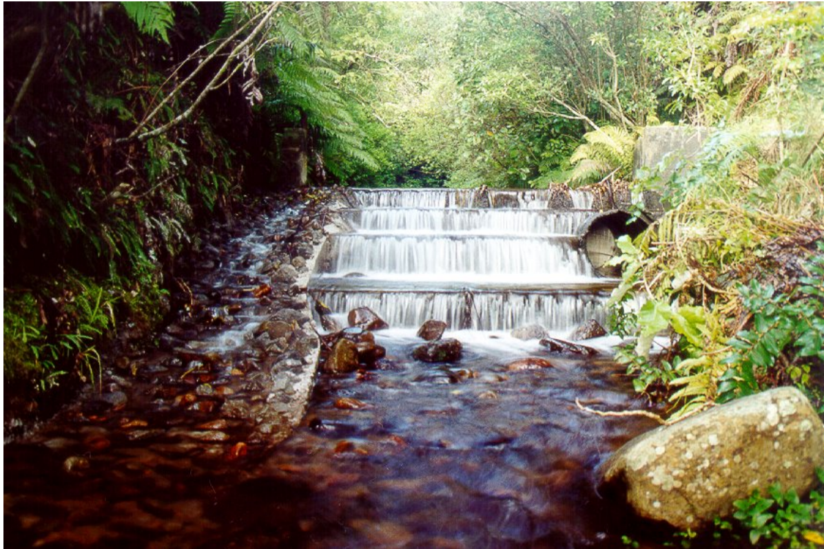
Photo 1 Wairau Stream weir and fish pass
