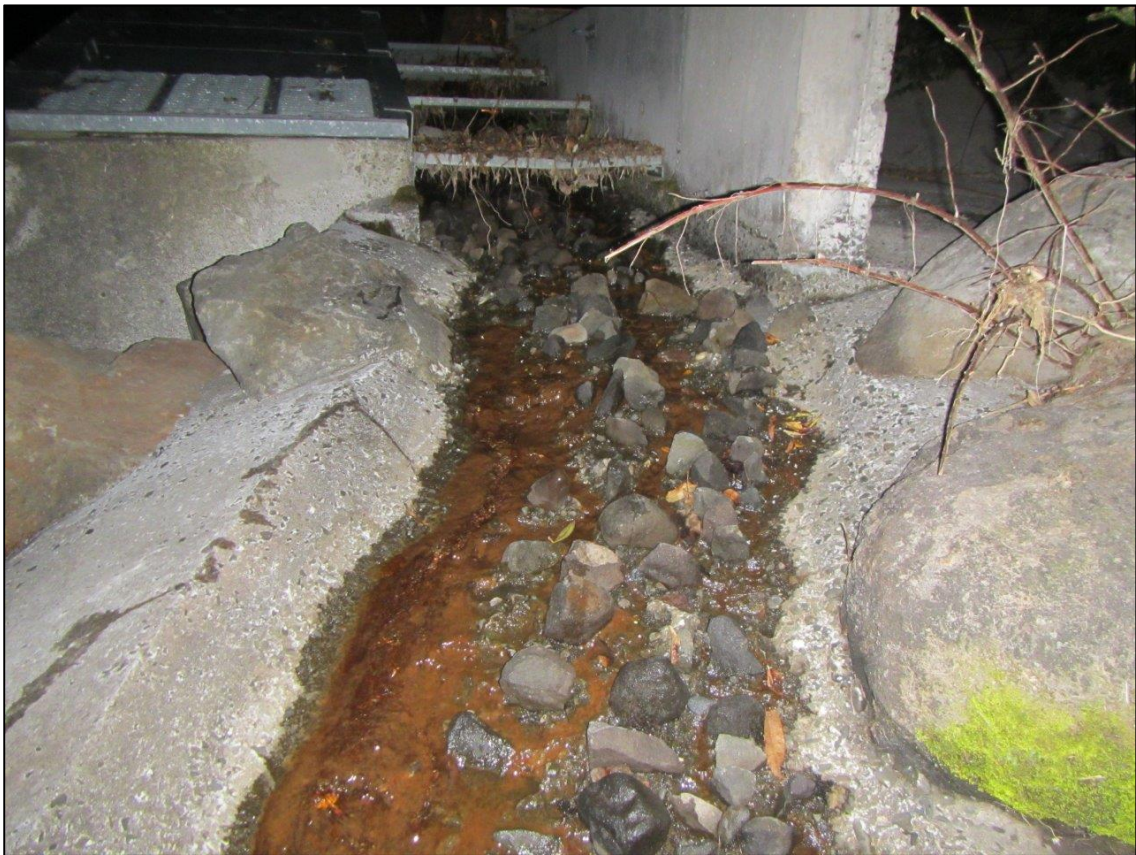
Photo 4 The fish pass with minimal flow, 20 April 2016.
