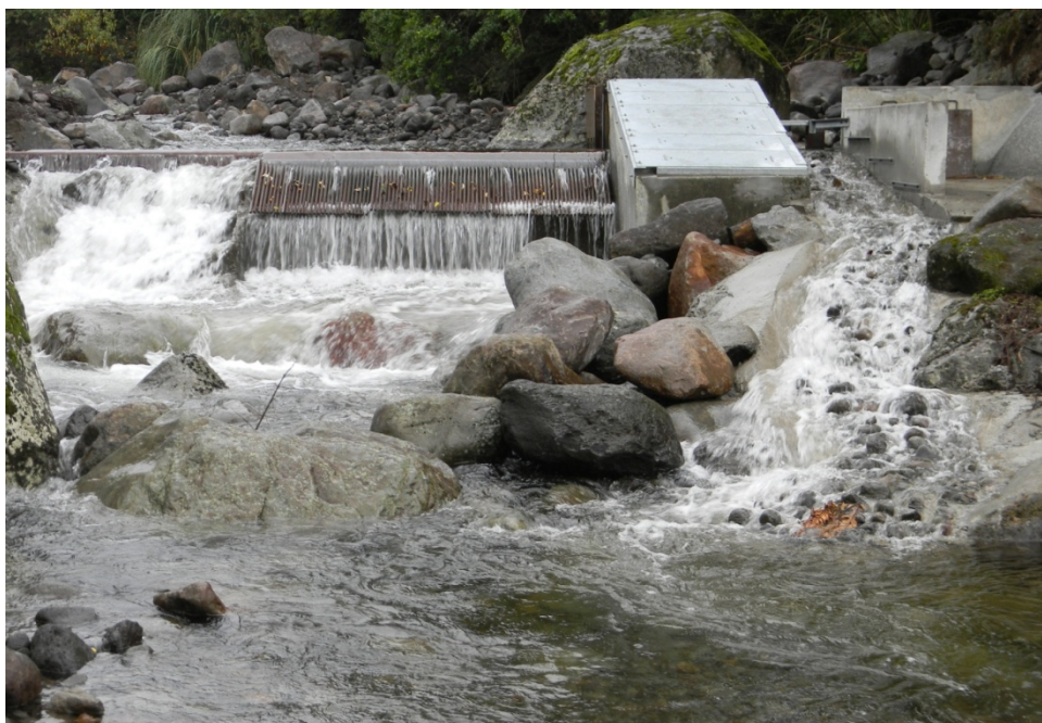
Photo 1 The upgraded Otakeho Stream weir, 6 May 2011.
