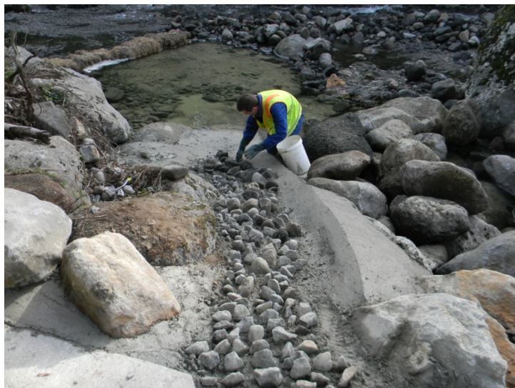
Photo 2 TRC biologist placing rocks in the steepest section of the new fish pass
