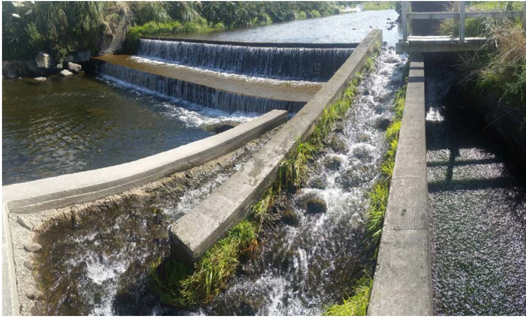
Photo 1 Oaonui Water Supply weir and fish pass, March 2016
