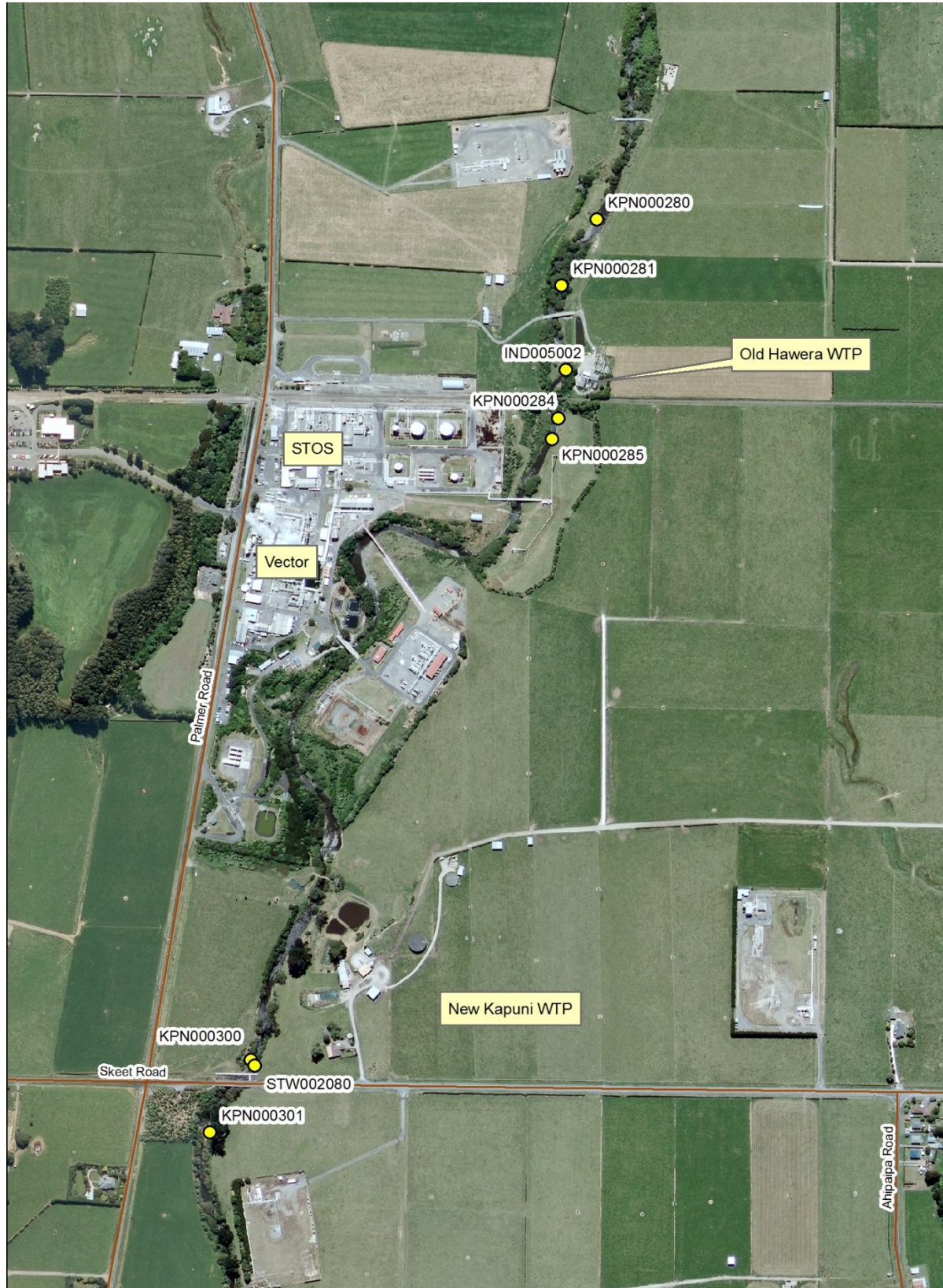
Figure 1 Aerial photo showing the location of the old and new water treatment facilities, and relevant sampling sites.
