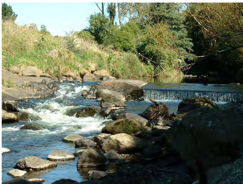
Photo 1 Waitara Water Supply weir in the Waiongana Stream
