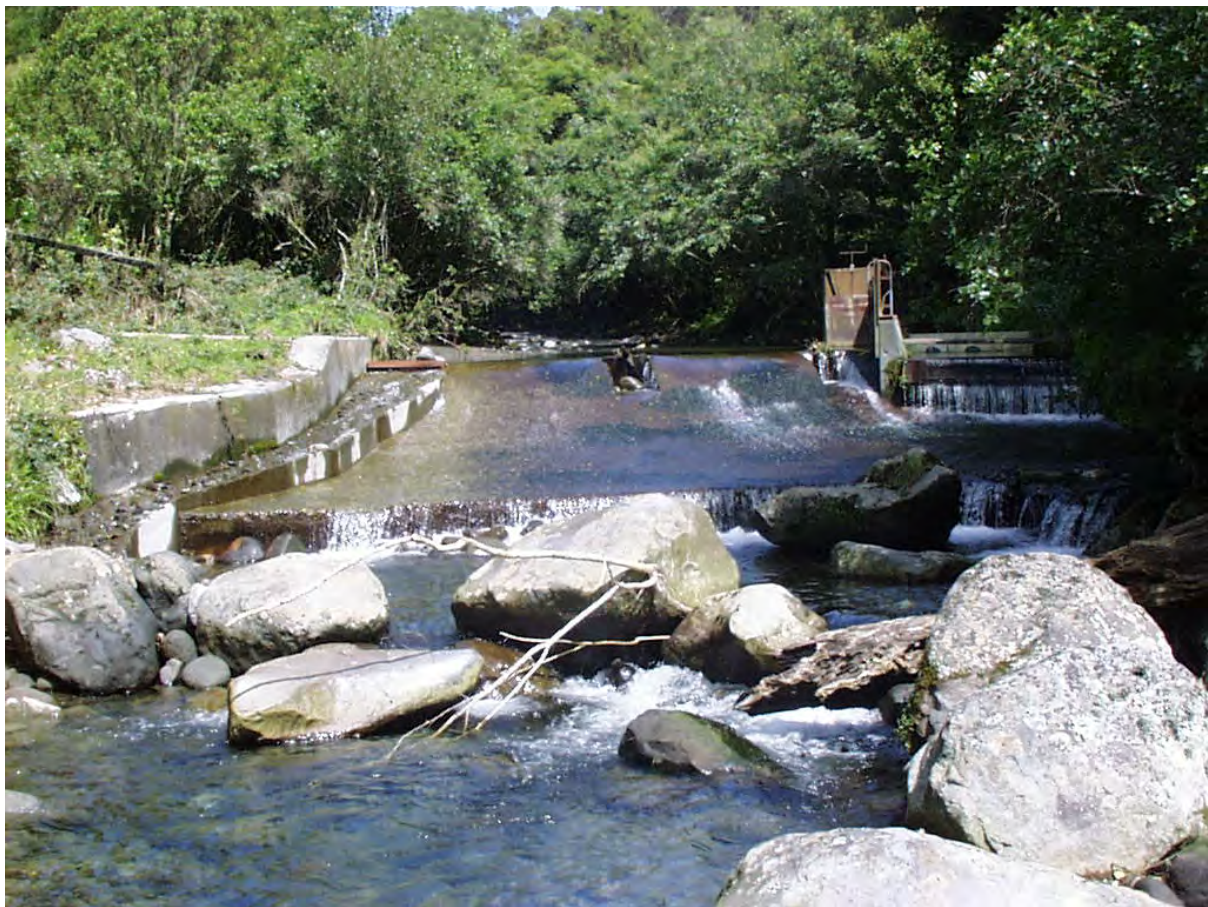
Figure 2 Ngatoro Stream weir and fish pass
