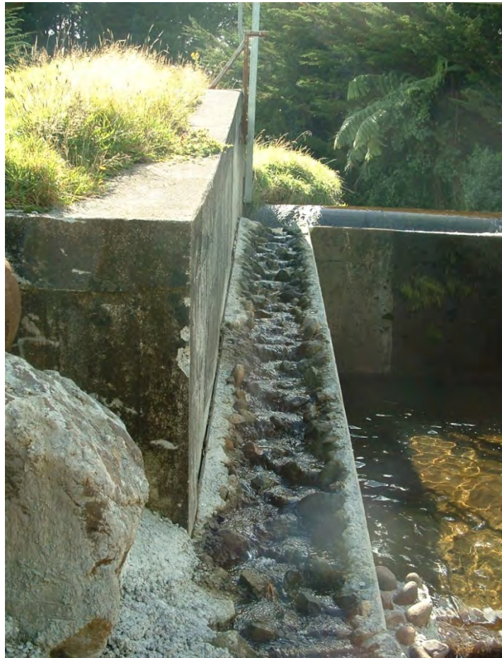
Photo 2 Fish pass on STDC weir in the Mangawheroiti Stream
