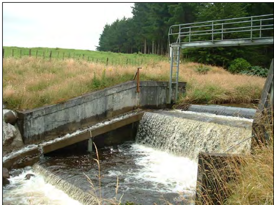
Photo 1 Mangawheroiti Stream weir and fish pass
