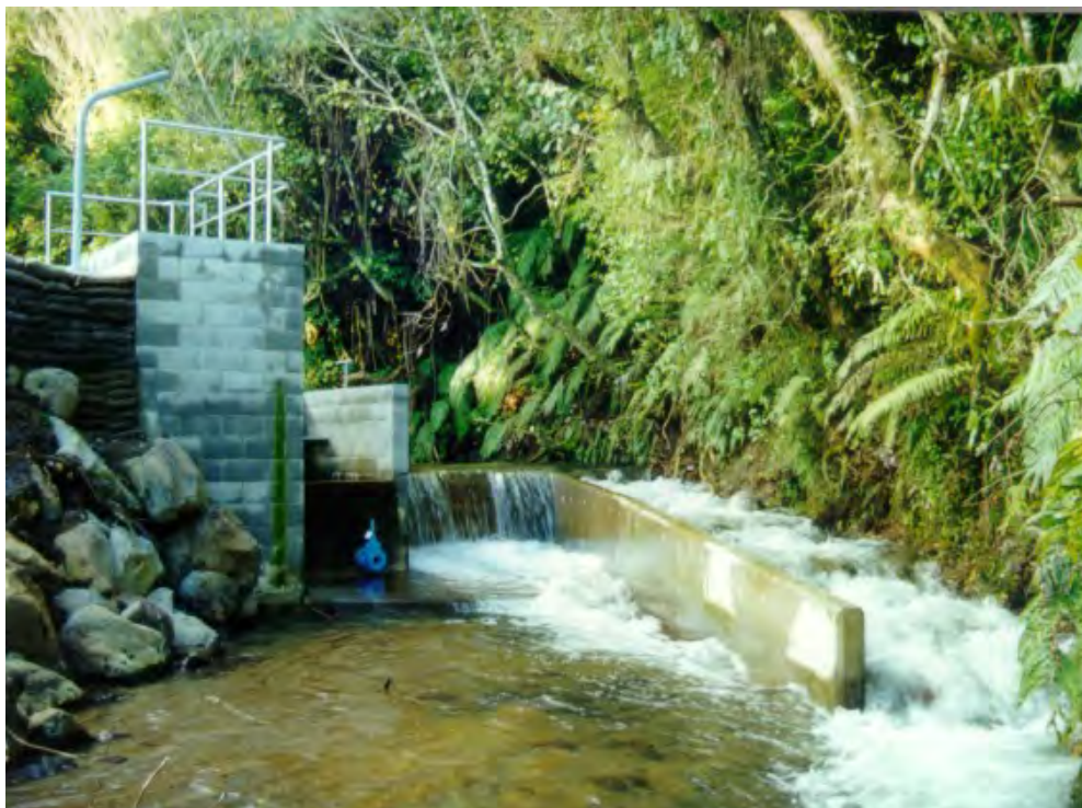
Figure 1 Weir downstream of Upper Palmer Road, in the Mangatoki Stream
