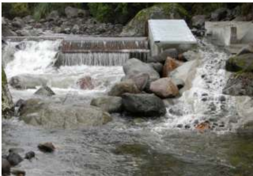
Photo 1 The upgraded Otakeho Stream weir, 6 May 2011.
