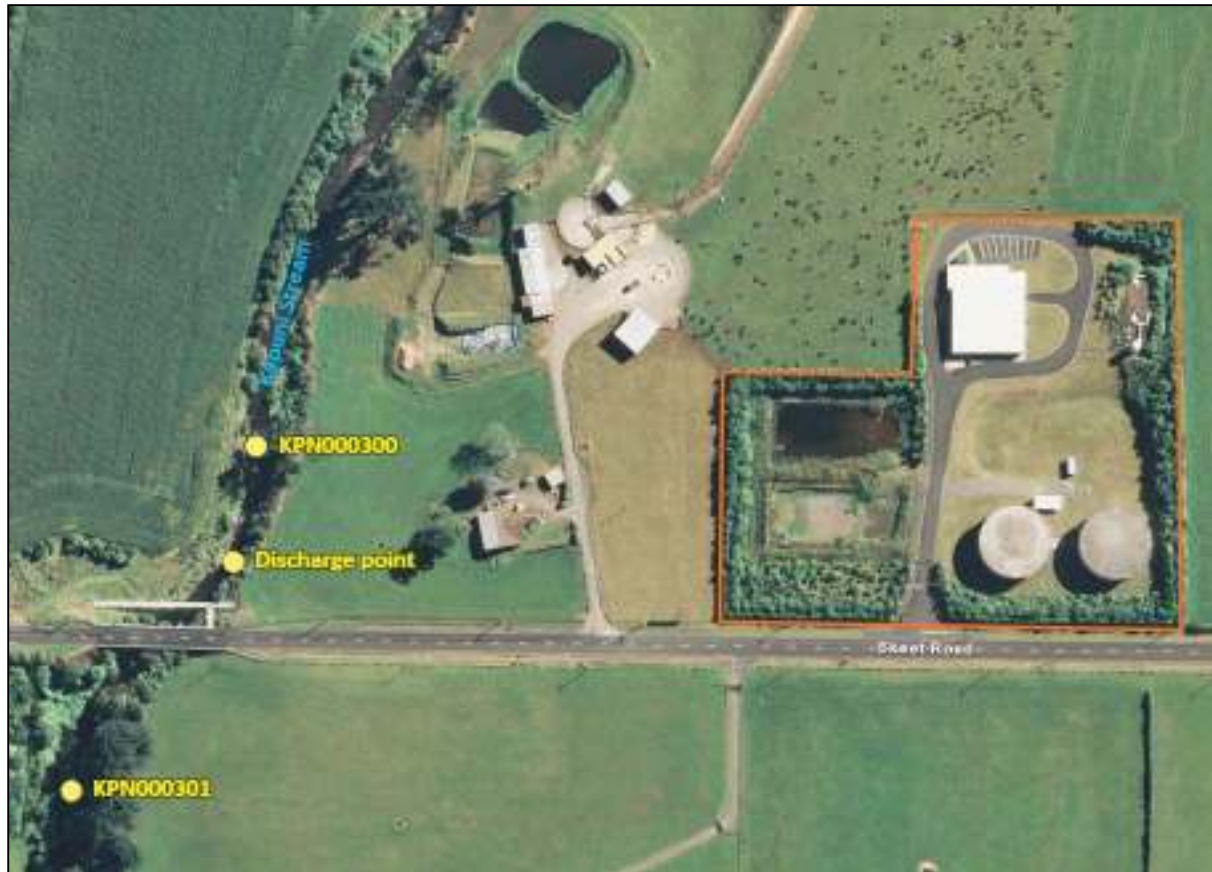
Figure 1 Aerial photo showing the location of the water treatment facility, and relevant sampling sites.
