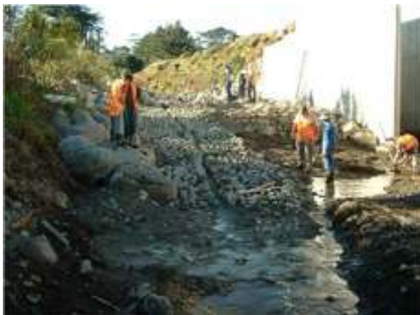
Photo 1 The STDC fish pass being installed September 2009
