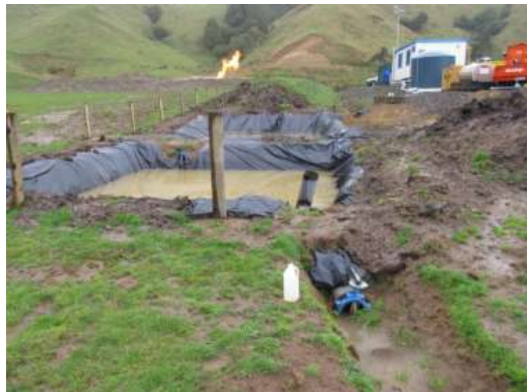
Photo 1 Wellsite flare (background) and skimmer pit (foreground), and discharge sampling
