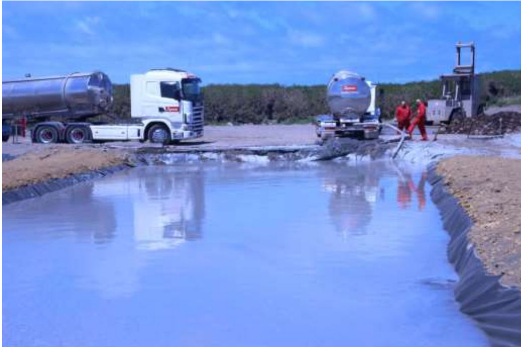
Photo 12 Oeo drilling waste land farm – lined mud storage pit
