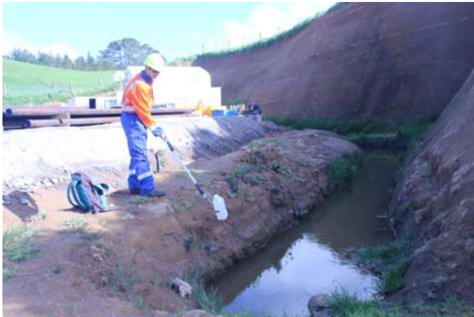
Photo 13 Cheal B wellsite – sampling wellsite drainage
