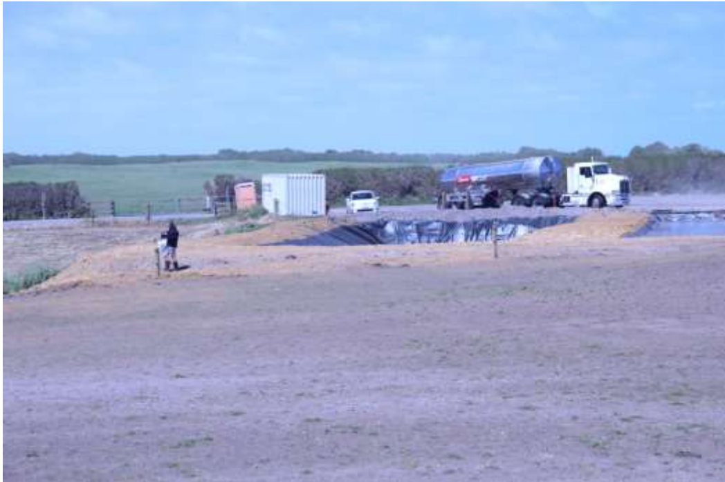
Photo 10 Oeo land farm – lined waste storage pits and soil sampling
