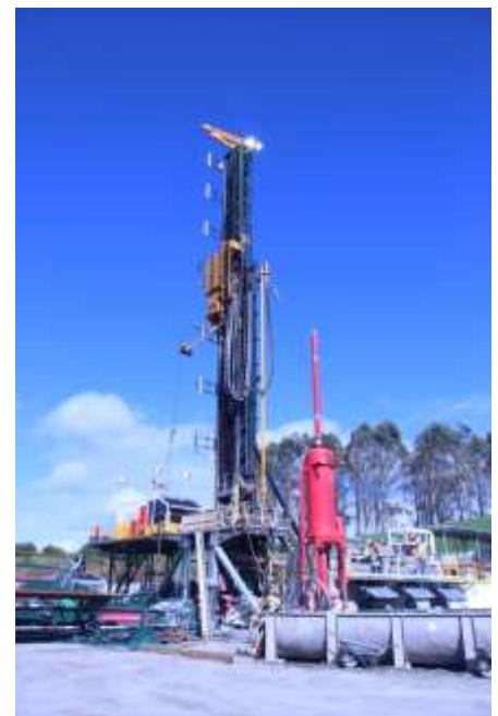
Photo 3 Cheal B drilling rig November 2012
