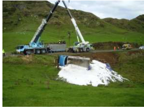
Spill of urea from a vehicle accident on State Highway 3
