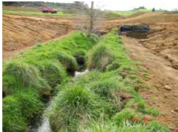
Figure 15: Unnamed tributary pre-realignment
