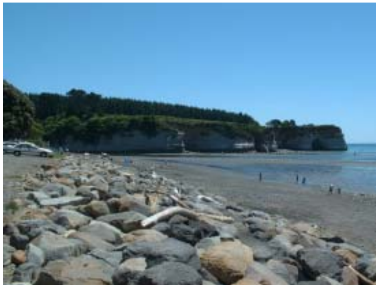
Urenui Beach – coastal erosion protection works
