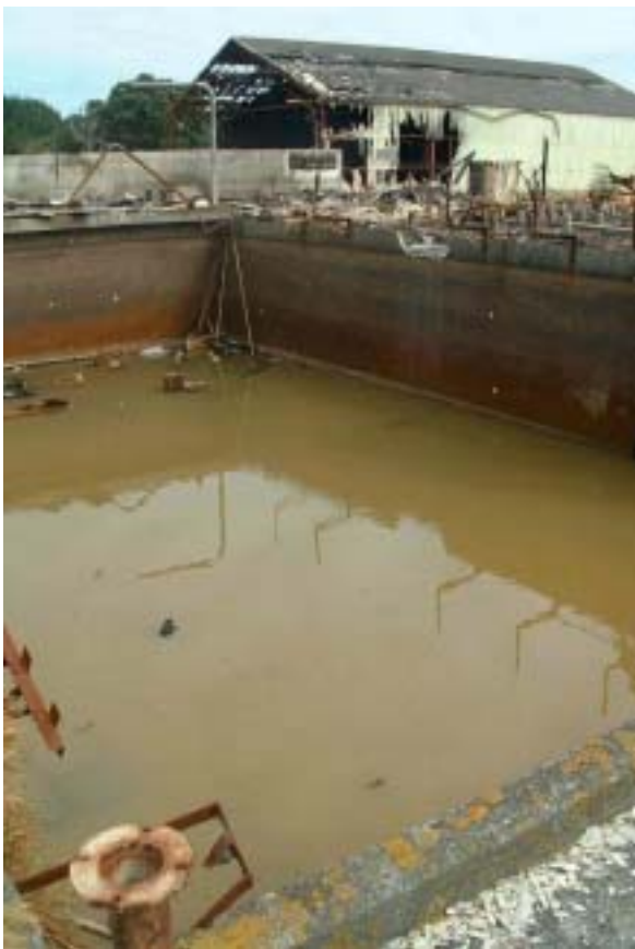
Photograph 2 Main Reservoir and Storage building (prior to preparation as containment facility)
