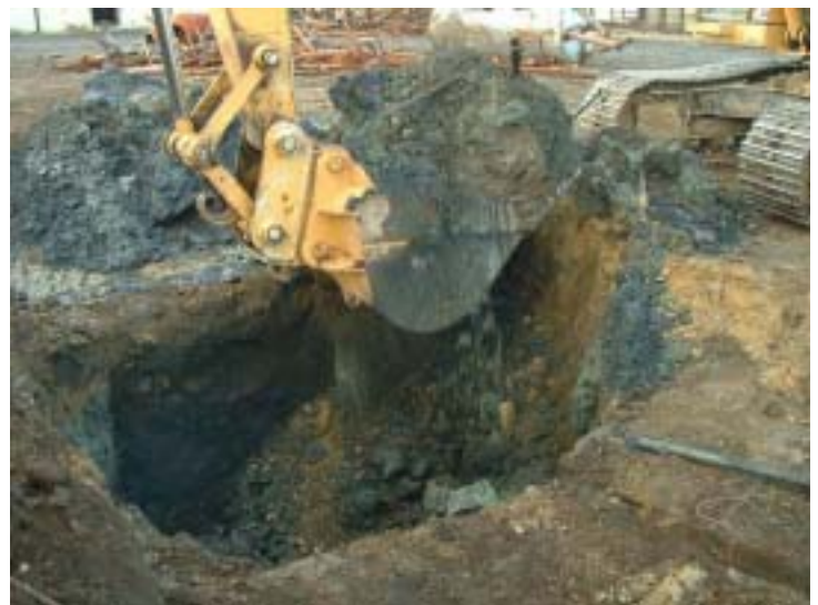
Photograph 5 Excavation of contaminated soil
