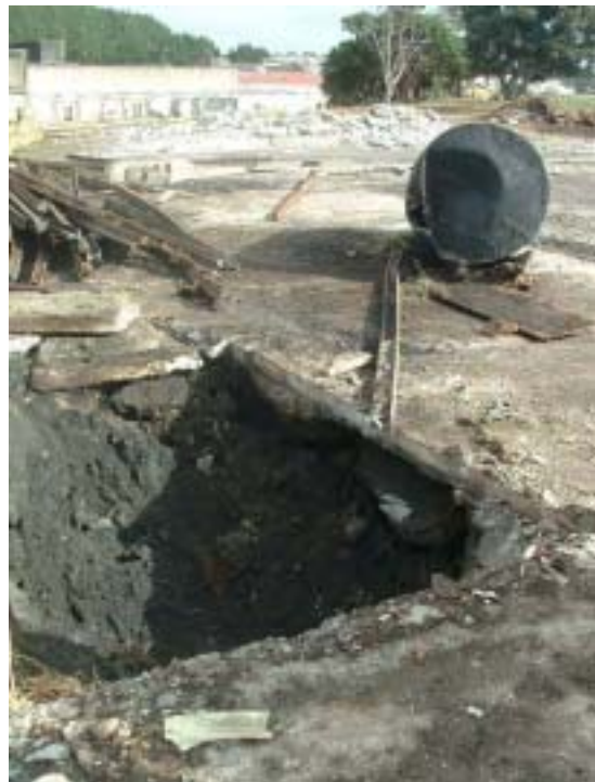
Photograph 3 Covered Unloading Platform tank and pit
