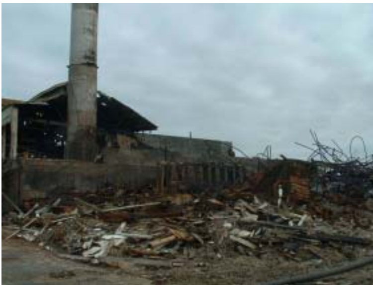
Photograph 1 Remains of the Freezing and Cold Storage Buildings
