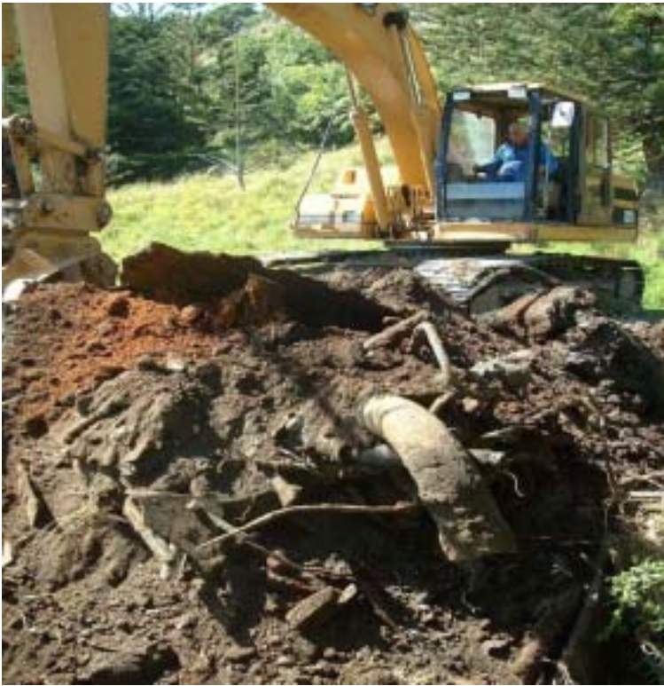
Photograph 11 Test pit spoil
