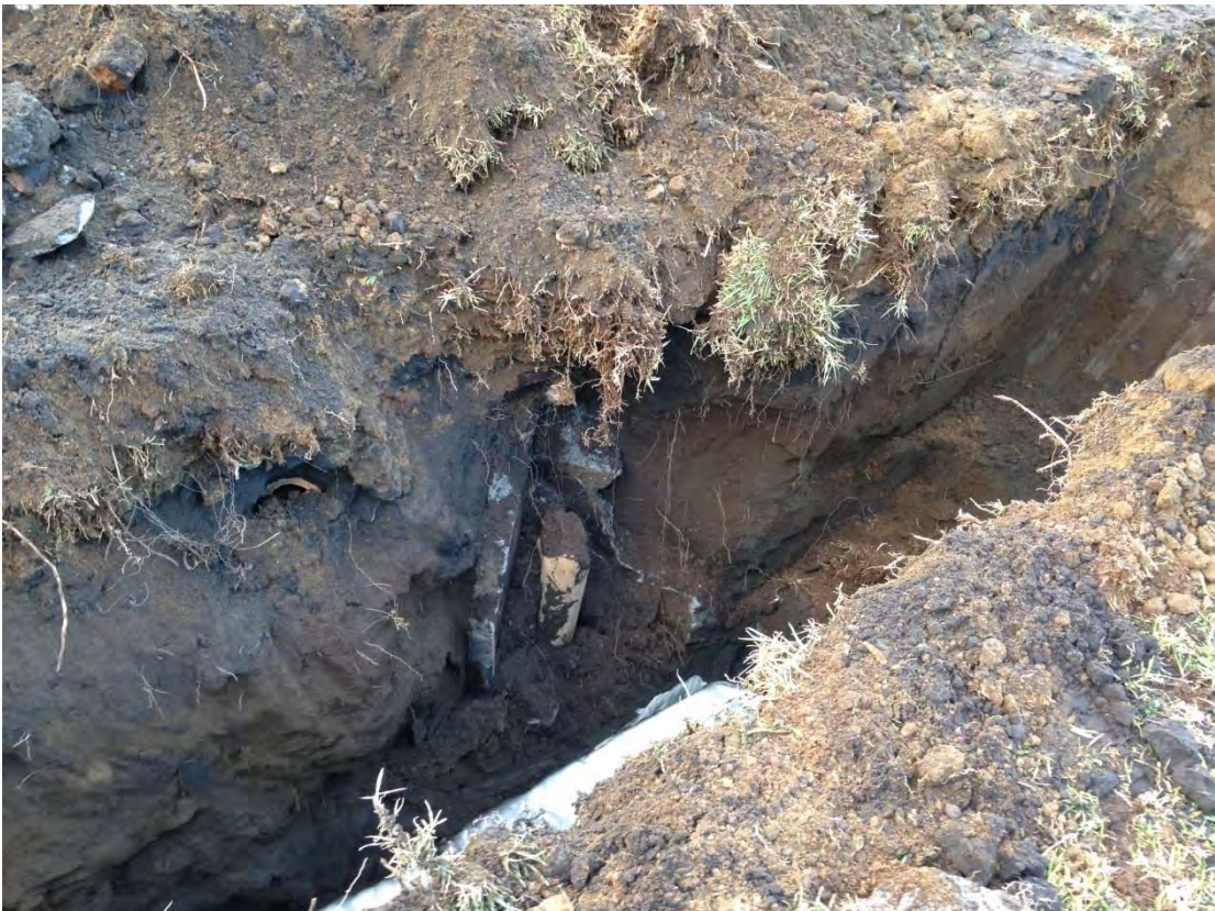
Photograph 12: Remnant building foundation encountered during the Marae investigation (SS20).
