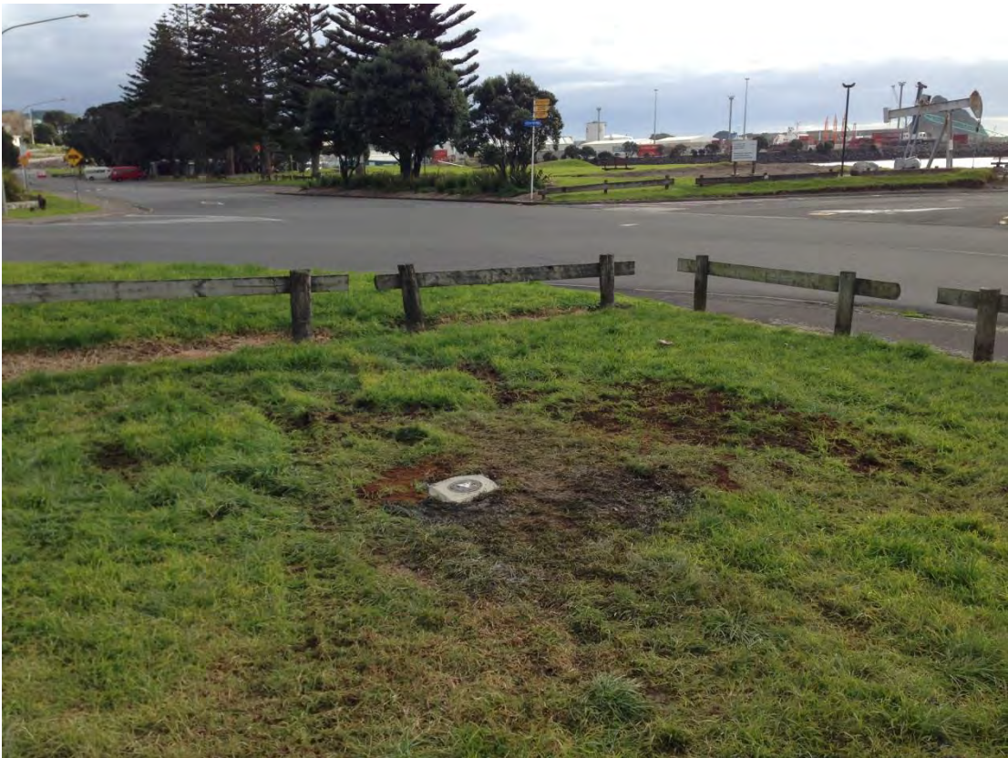
Photograph 8: View of completed monitoring well (MW1).
