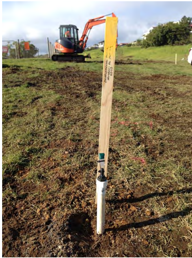
Photograph 9: View of ground gas monitoring point installation.
