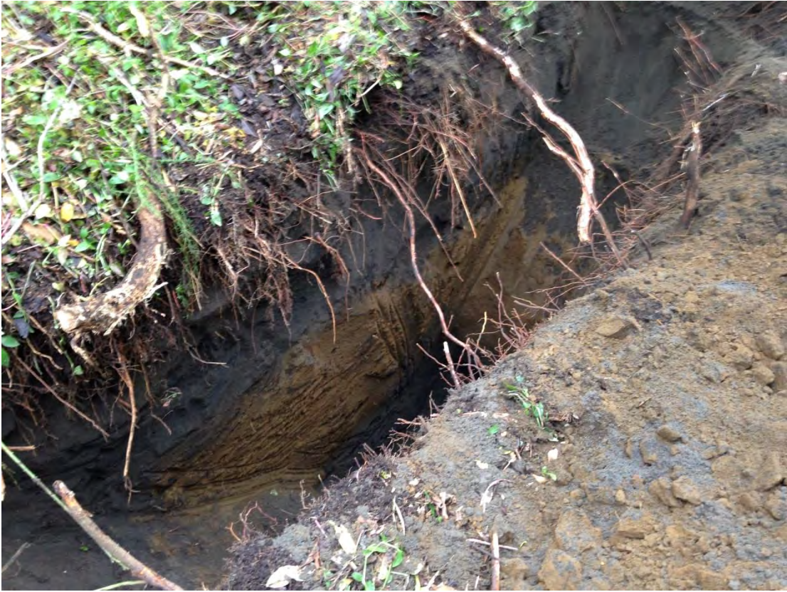
Photograph 17: Test pit excavated during the Moturoa 3 oil well investigation.
