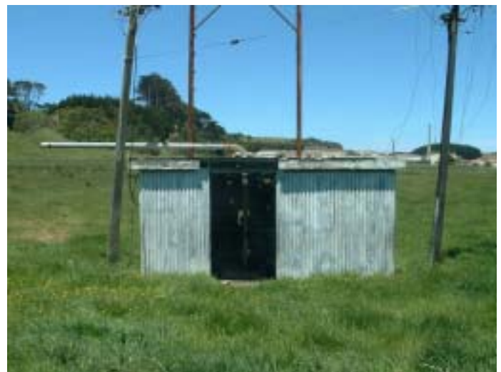
No. 7 well pumpshed and factory to south
