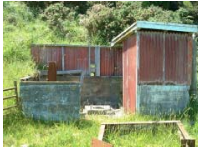
No. 4 artesian well pumped
