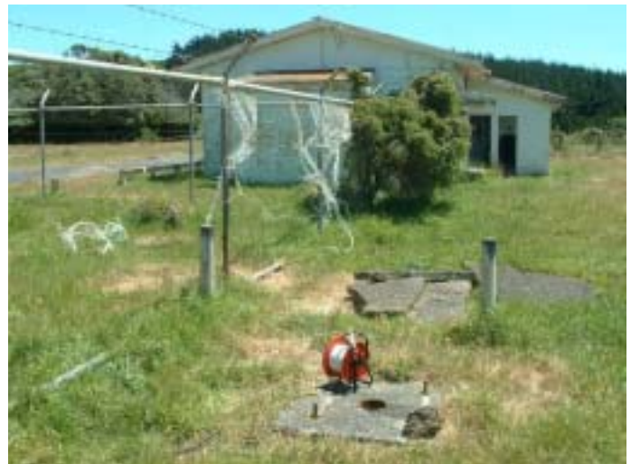
No. 3 artesian well & butchers shop to west
