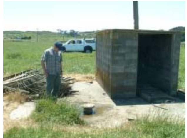
No. 6 well and pumpshed
