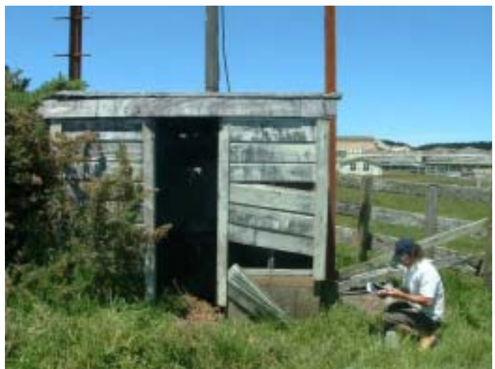
No.1 well pumpshed, with factory to south
