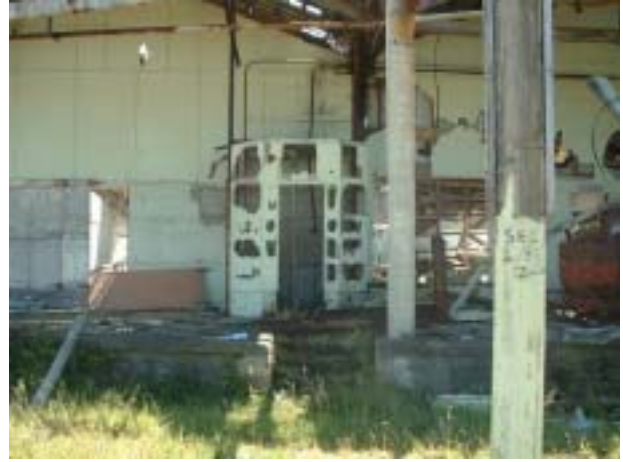
No. 2 well location
