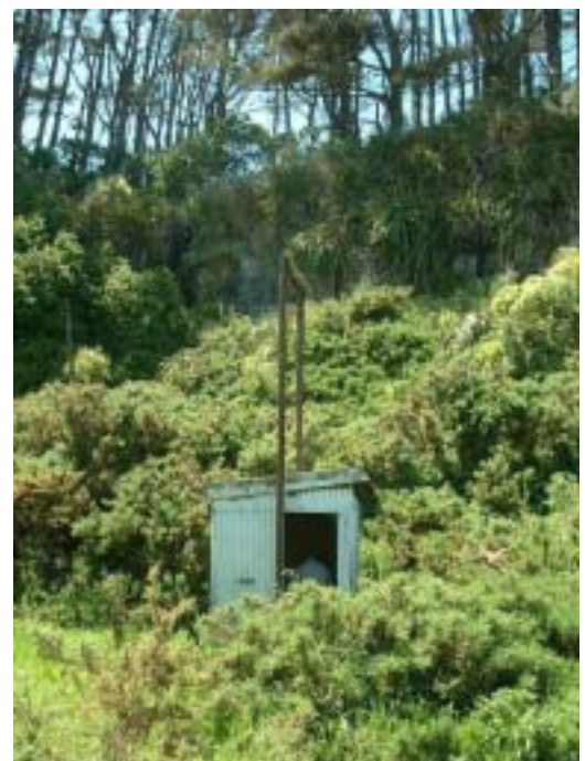
No. 5 artesian well pumped
