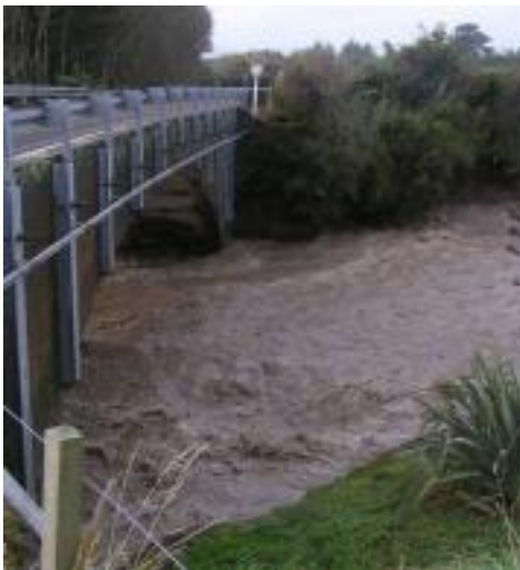
Photo 5 Stony River SH45 bridge, flood flows of about 200 cumecs
