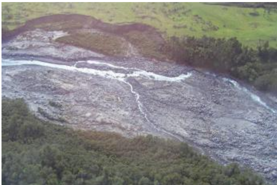
Photo 4 Stony River – Vicinity of Egmont National Park boundary – bank erosion
