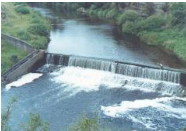
Photo 13 Kaupokonui Stream Weir build for dairy factory water supply at Glenn Road
