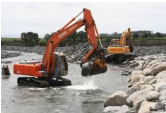
Photo 15 Stony River – Heavy rock training work to divert channel into new alignment
