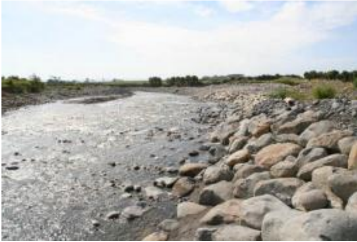
Photo 16 Stony River – Completed diversion and new channel to mobilise and increase gravel movement and reduce deposition
