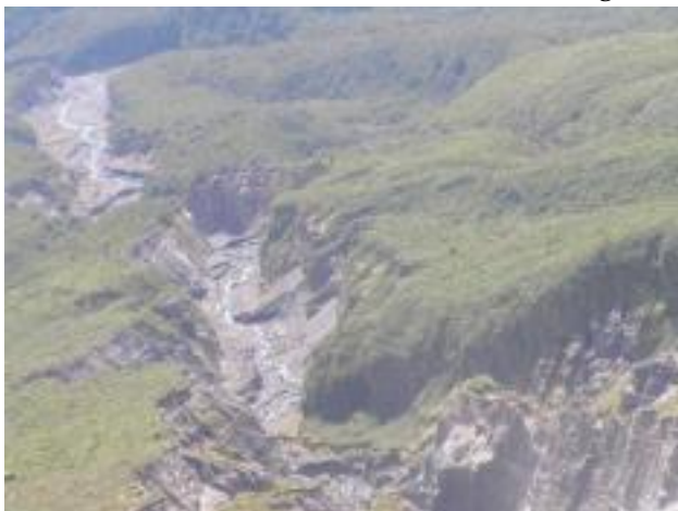
Photo 9 Pyramid Stream. Erosion in upper catchment which discharges into Stony River within Egmont National Park
