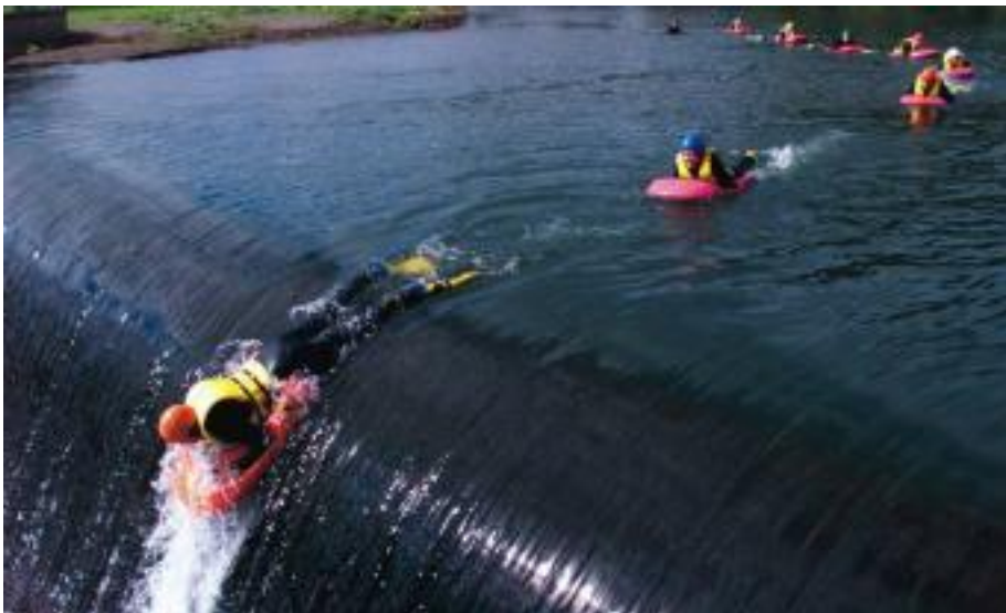
Photo 17 Dam dropping. Waingongoro River Normanby Weir diversion for electricity generation
