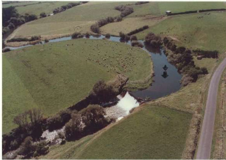
Figure 13: Existing Dam on the Waingongoro River (source: BECA 1985)
