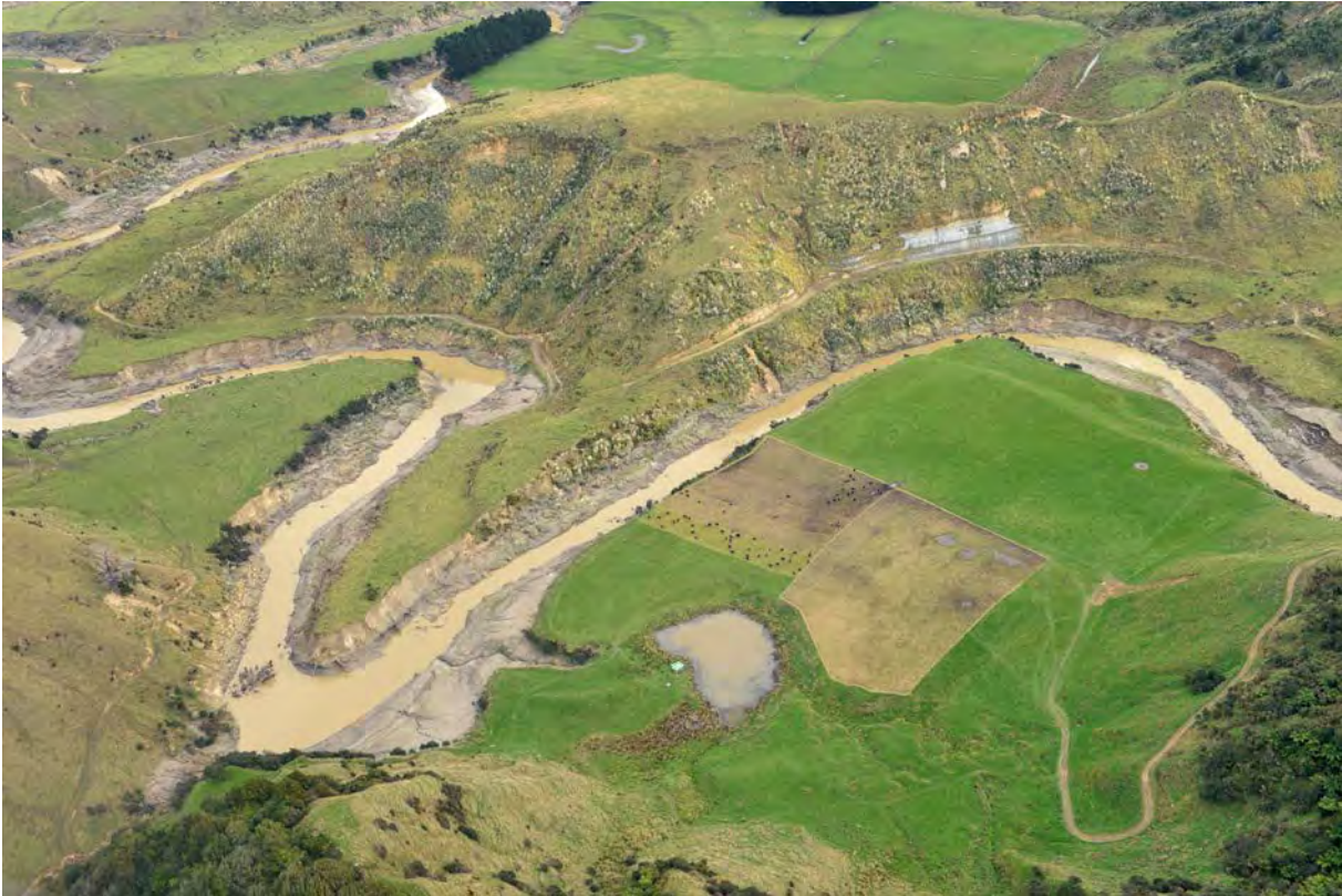
Figure 51 Severe streambank erosion along the lower reaches Whenuakura River, near Patea. (GNS Photo: D02_2930)
