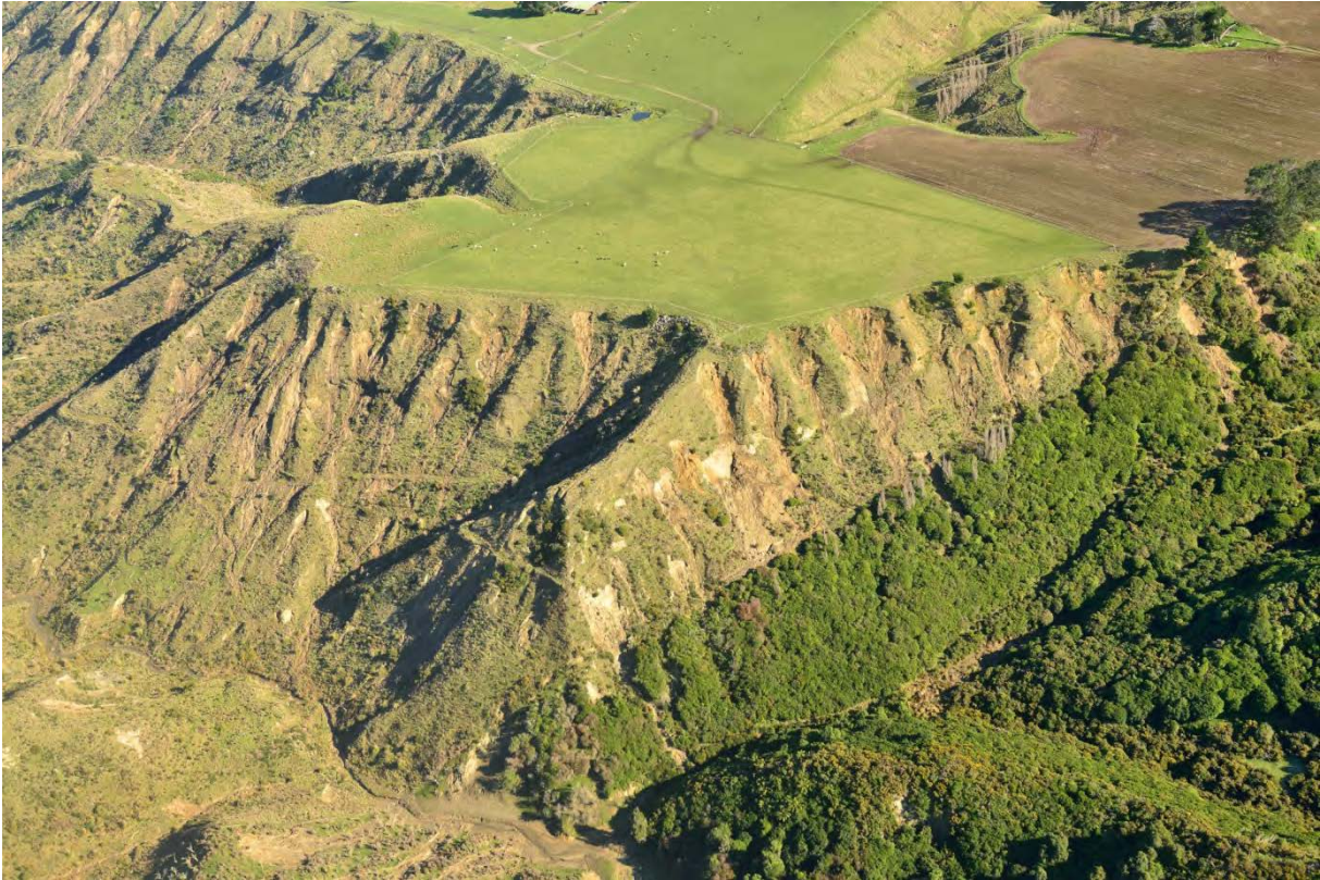
Figure 25 Severe landsliding in head of Matarawa Stream, north of Fordell. Note location of landslide initiation at terrace-scarp boundary. (GNS Photo: D02_1496)
