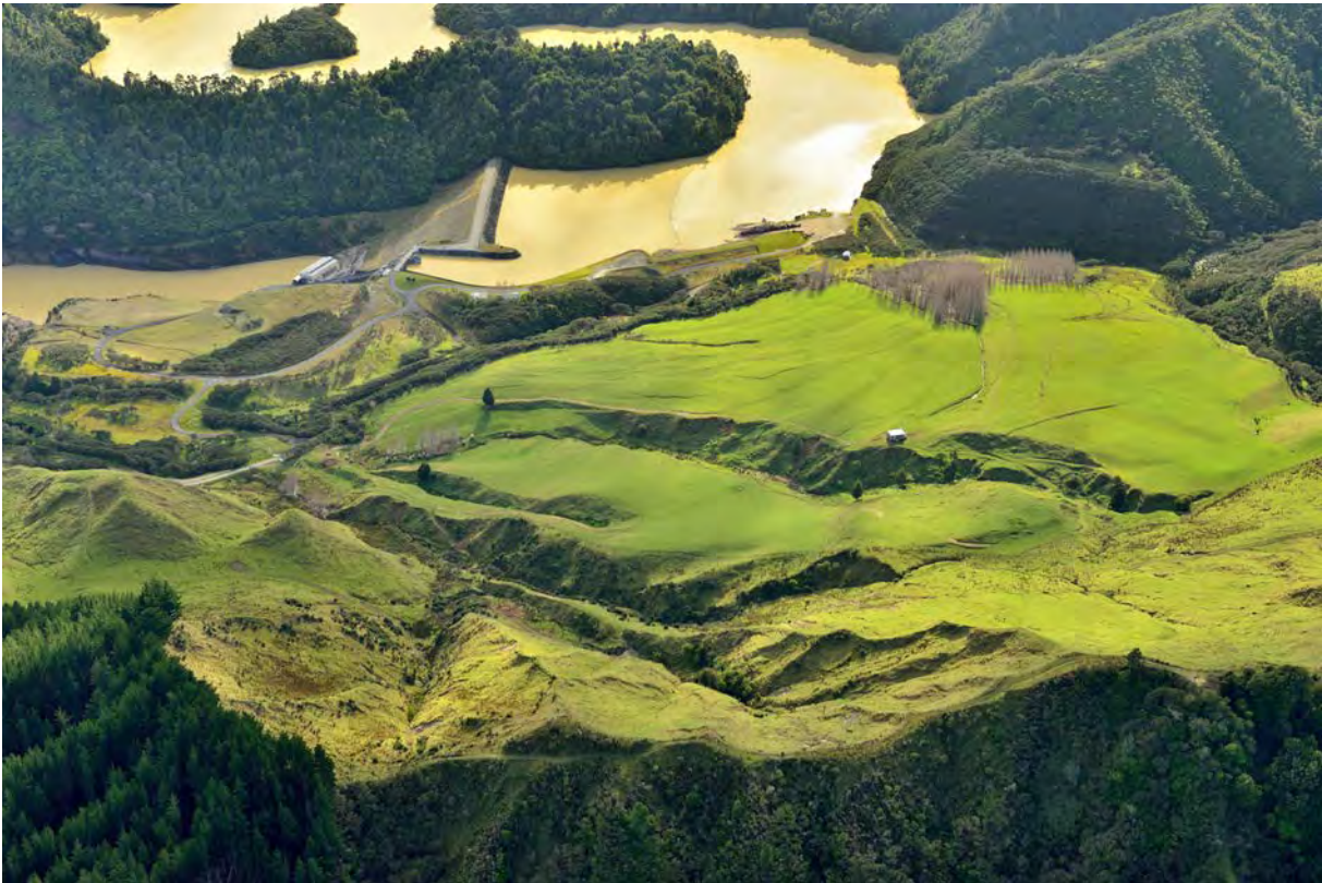
Figure 53 The Patea Dam, and an ancient deep seated landslide to the centre right. Note pre-existing signs of movement on the landslide (cracks). However, it was not possible to determine whether the rainstorm had caused movement of the landslide. (GNS Photo: D02_2856)
