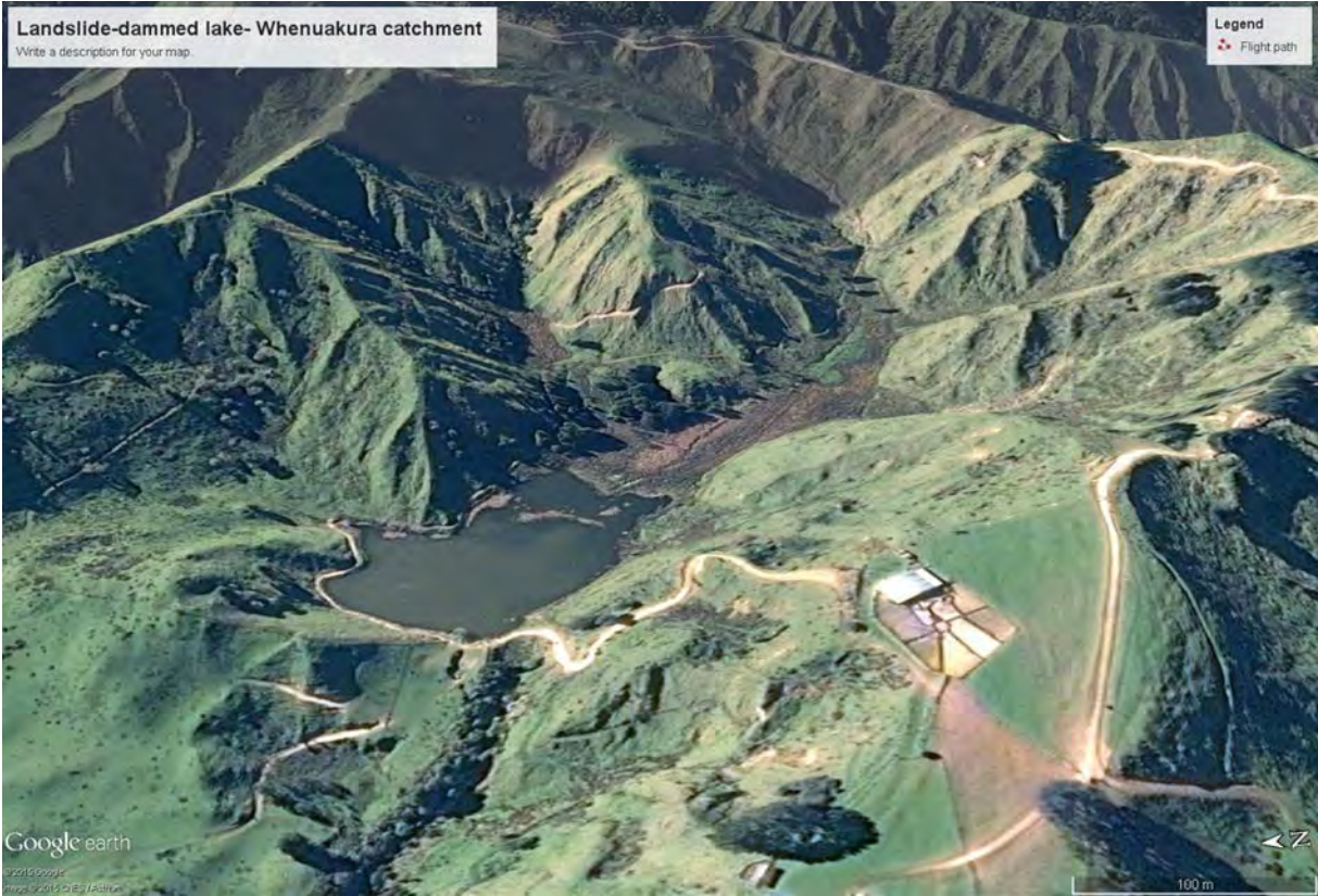
Figure 59 Google Earth image (September 2013) showing lake, outlet and access track prior to failure.
