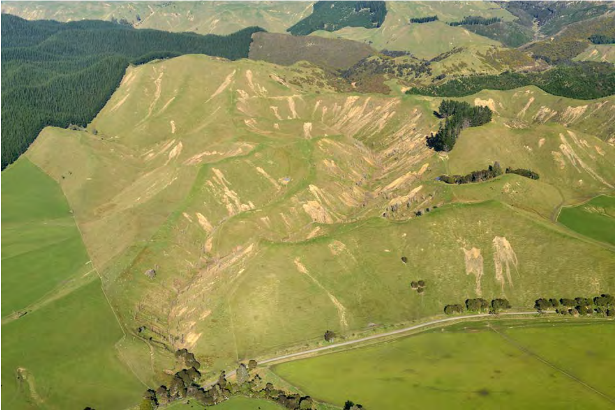
Figure 13 Severe landsliding (centre of photo) within area where landsliding has been classified as moderate. Turakina Valley near Lakes Ngaruru and Namunamu. (GNS Photo: D02_1708)
