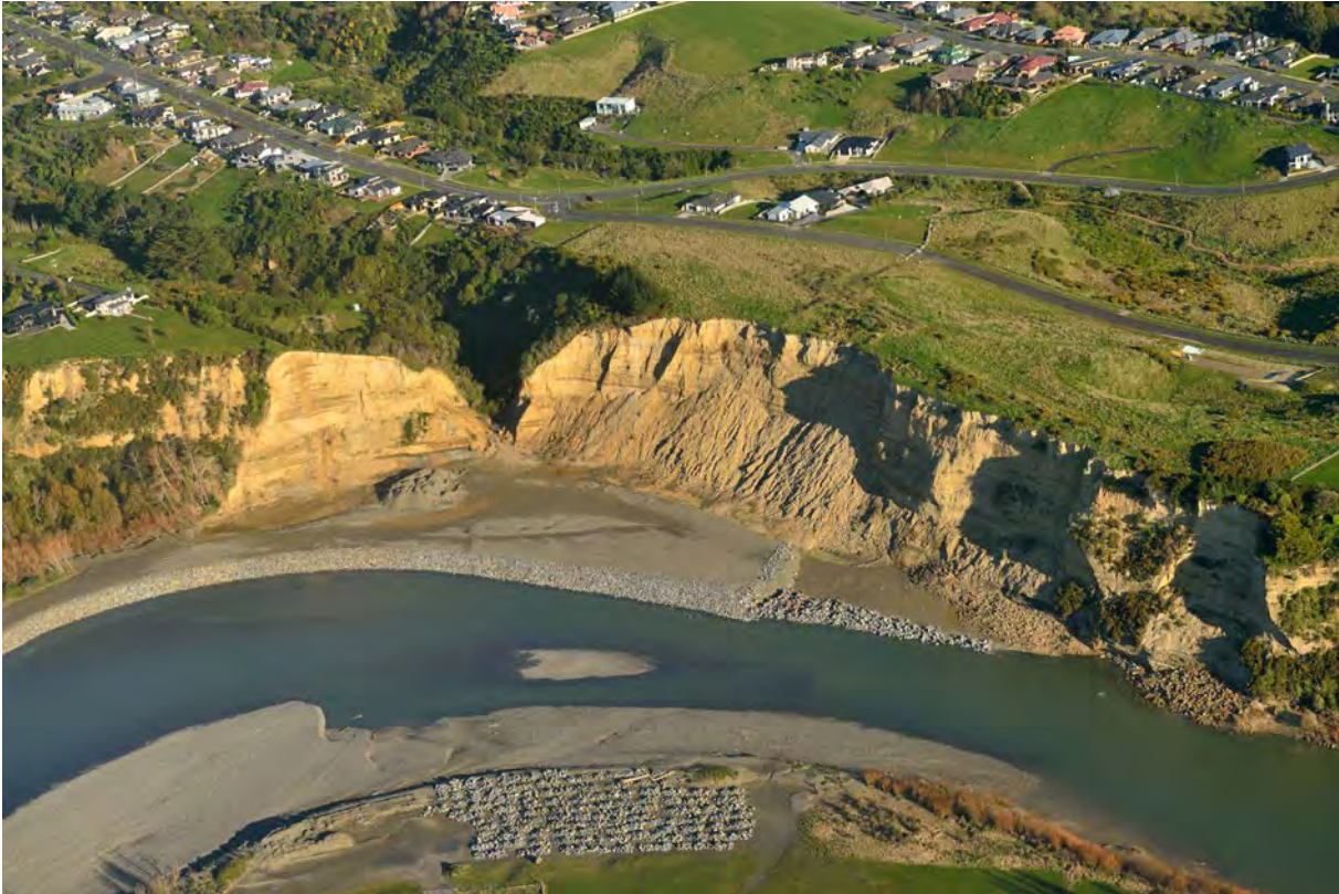
Figure 36 Cliff failure along the Manawatu River at Anzac Park, Palmerston North. (GNS Photo: D02_2080)
