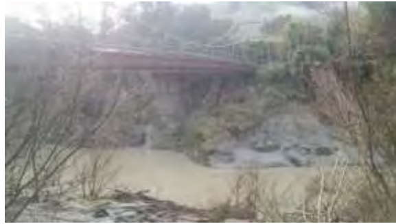
Photo 28: Rimunui Station bridge, Upper Waitotara Valley Road
