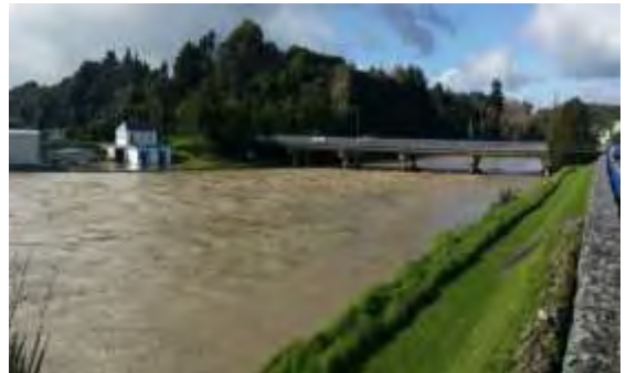
Photo 24: Waitara River at Bridge
