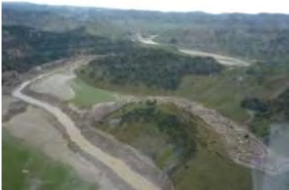
Photo 1: Waitotara River / Werewereonga Stream showing effects of Lake Mangawhio culvert failure
