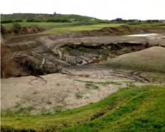
Photo 33: Flood damage at the McColls
