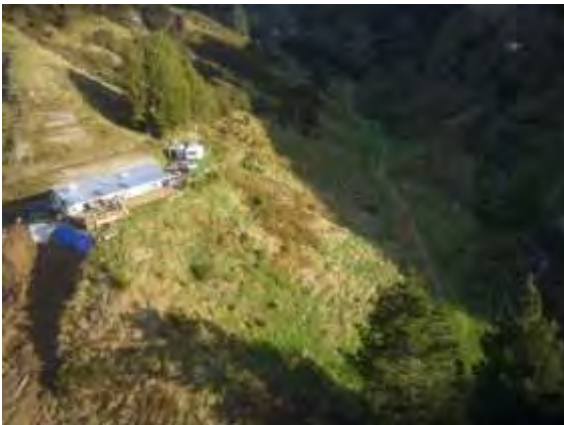
Photo 14: Okoki Rd, slip threatening Crawford property
