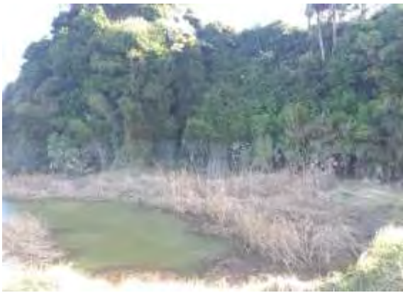
Photo 20: Waitara River bank damage below SH3
