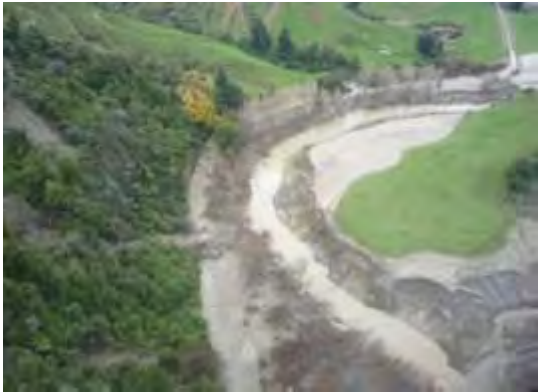
Photo 5: Road closure & silt on Waitotara Valley Rd
