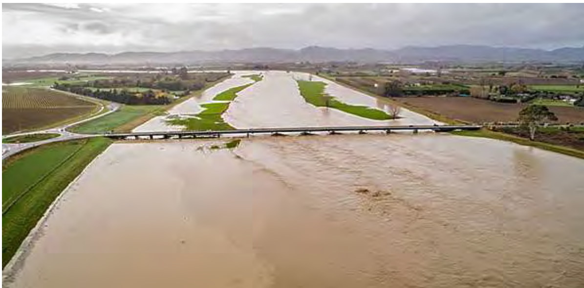
Waipaora River stop-banks containing 11 June 2018 flood event at State Highway bridge to Gisborne. NB Te Karaka township was cut off due to flood waters crossing the State Highway where there are no stop-banks.
