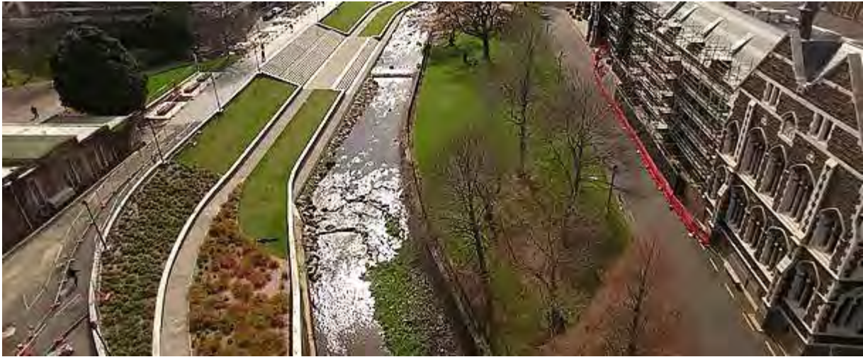
Water of Leith at University of Otago clock tower showing the amenity value achieved through sensitive design of river control and flood management works.
