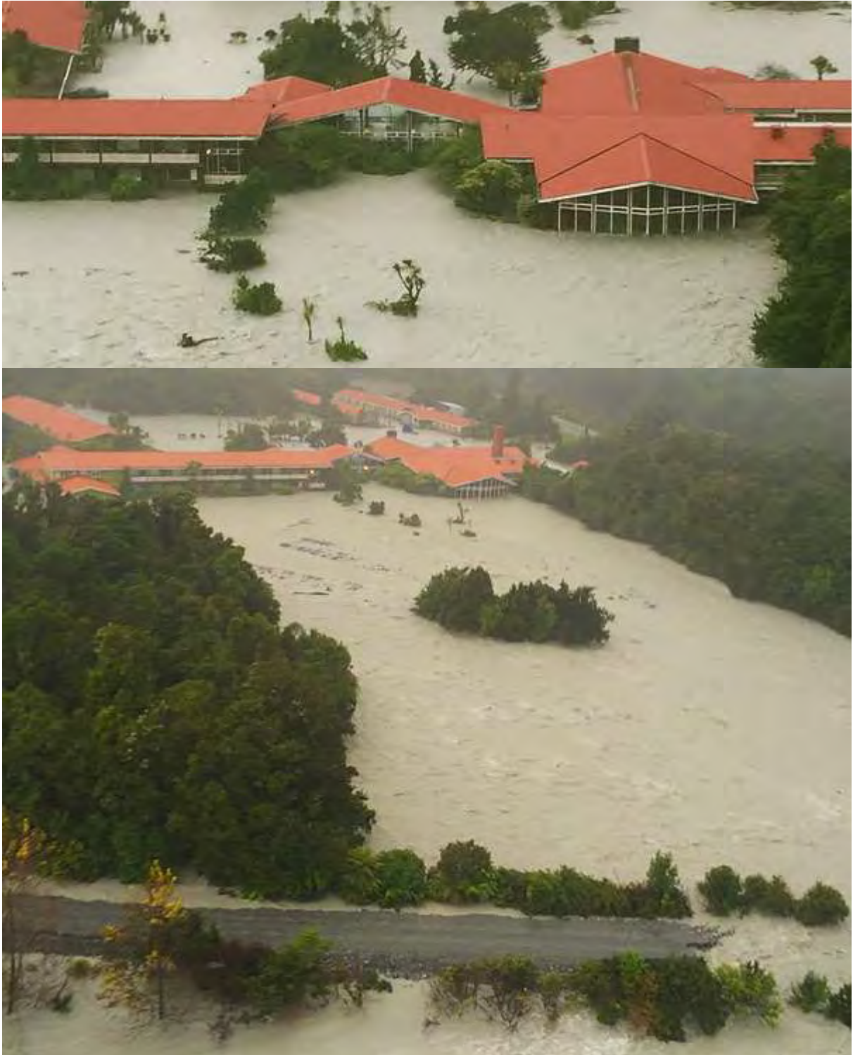
State Highway 6 was closed, and 70 staff and guests were evacuated from the Scenic Circle Hotel when the Waiho River breached its banks in March 2016.
