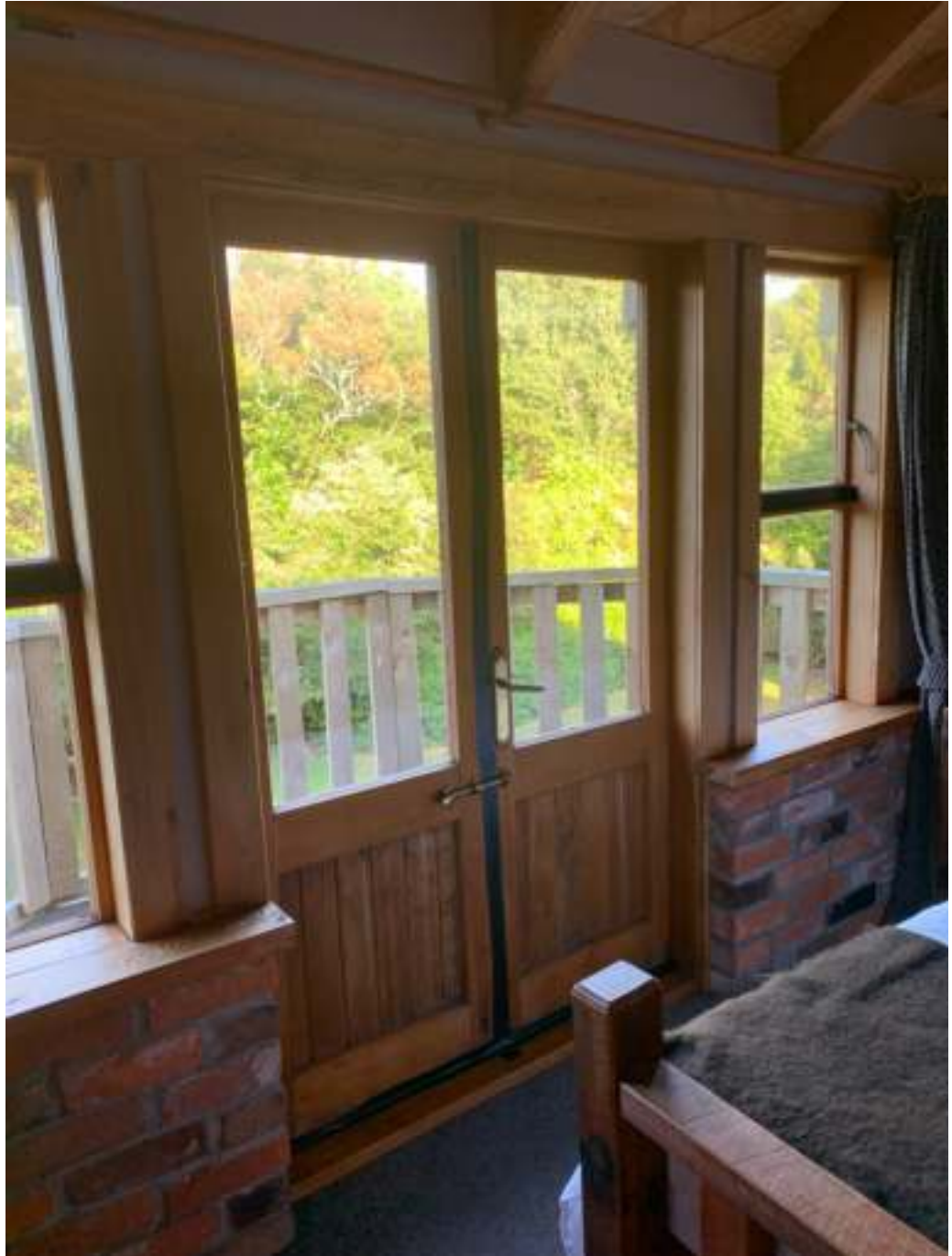
Photo 2: Our now abandoned, master bedroom with tape on doors and windows
