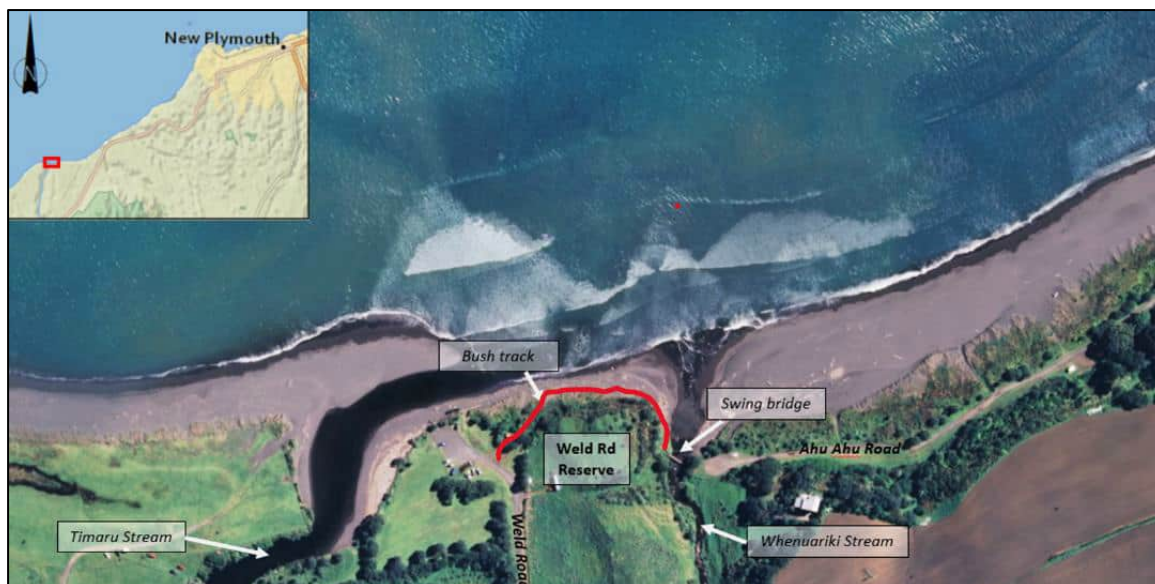
Figure 1.3: General outlined in red shows the pathway and rock revetment work taking place on the western side of the bridge replacement site (identified as 'swing bridge').
