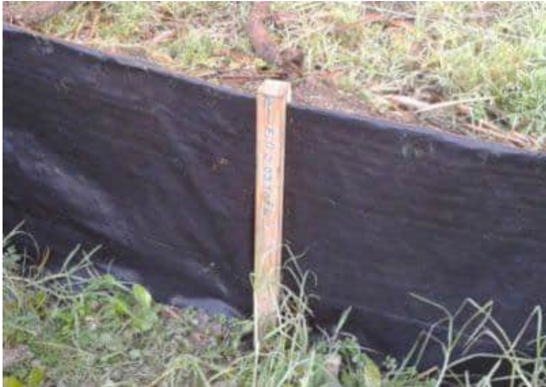
Battens joining silt fence fabric ends (Source: Southern Skies).
