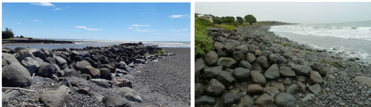
Figure 12 Photographs showing examples of colour, form and character of local rock revetment in context of beach and river environments.
