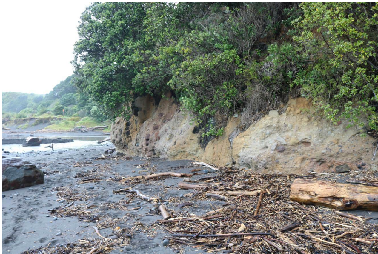
Figure 31 Photograph showing natural character and geological form of the headland cliff.
