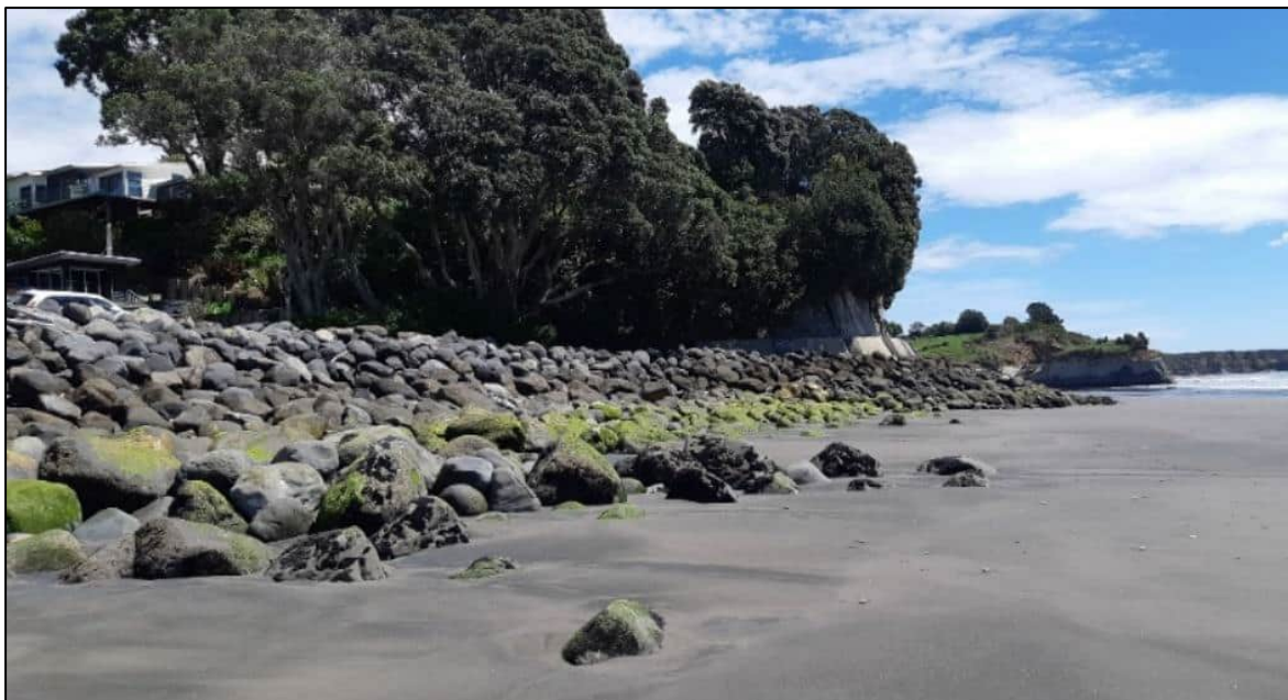
Figure 5.2 A similar style of rock revetment along a segment of the New Plymouth coastal walkway which appears visually integrated with the vegetated backdrop after aging. (Source: NPDC, 2022).
