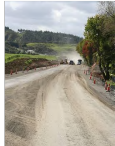
Construction of Awakino northbound passing lane
