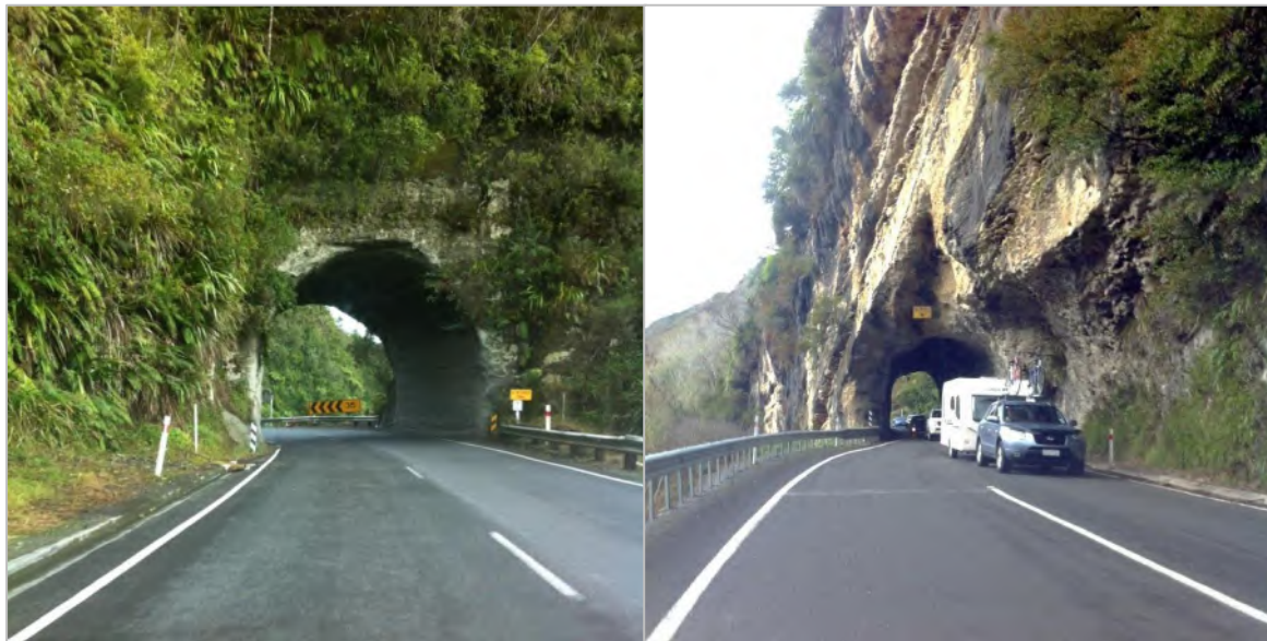
The two tunnels on the route – on Mount Messenger (left) and the Awakino Gorge (right), April 2014
