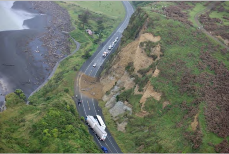
December 2009 slip on SH3 south of Mokau
