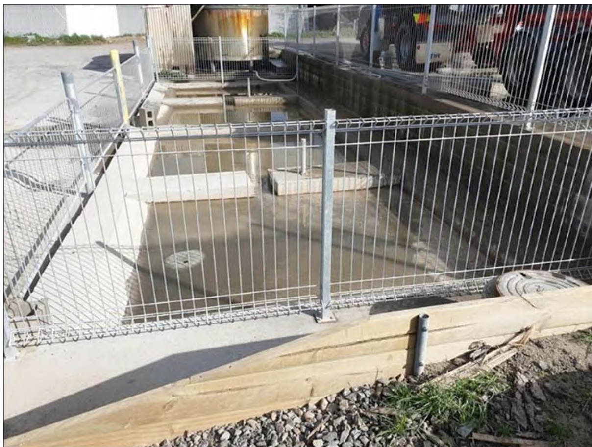
Photo 7 FBT truck wash discharge to trade waste
