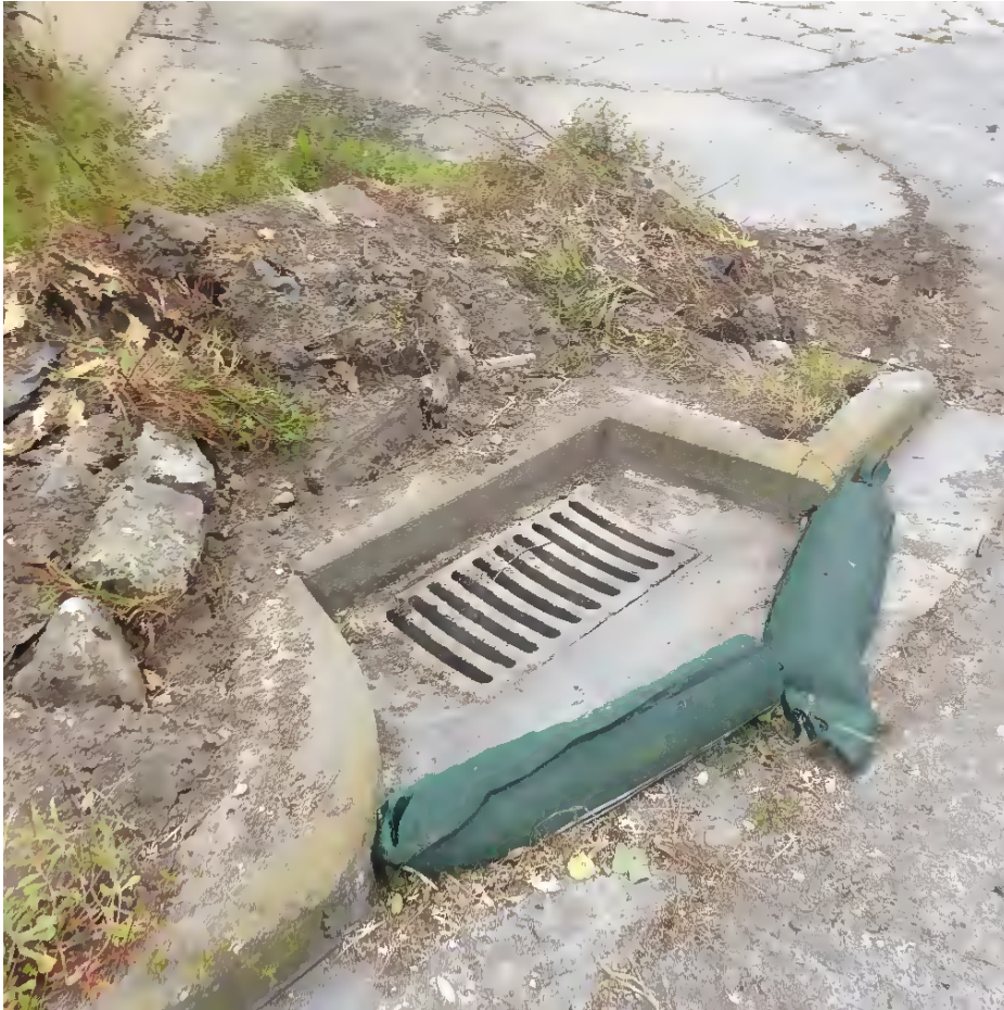
Photo 2 Bunding on stormwater drains, November 2021
