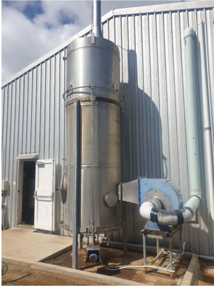
Photo 7 Zelam scrubber and associated bunding, September 2020
