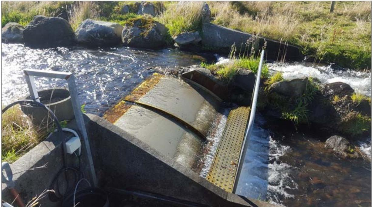
Photo 1 CCCWSL's weir and intake screen
