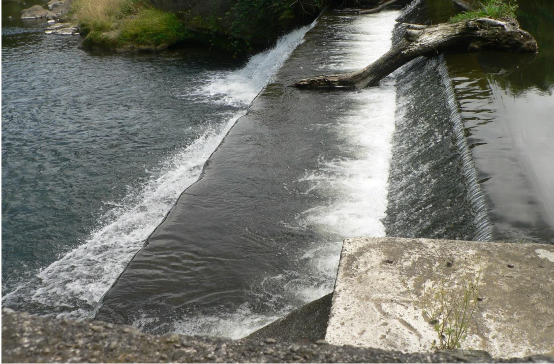
The Riverlands Eltham weir on the Waingongoro River that needs removing.
