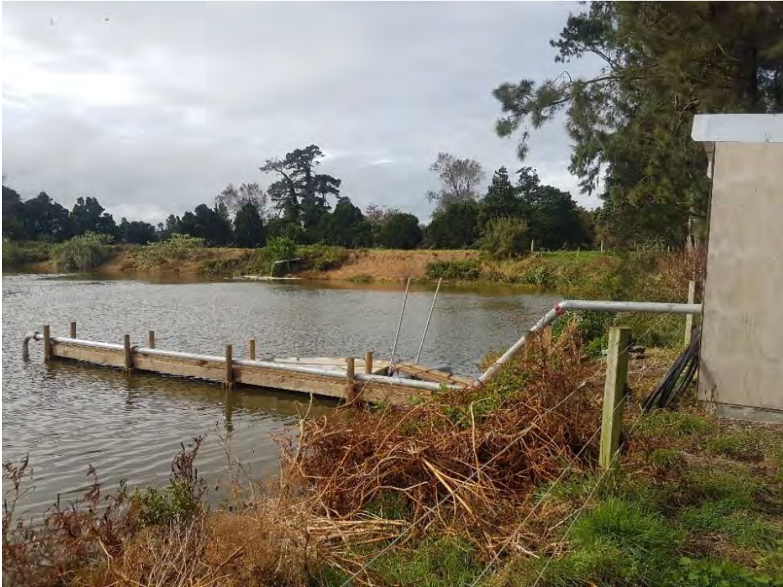
Figure 11 Pump systems from final aerobic ponds which transport effluent to the stream
