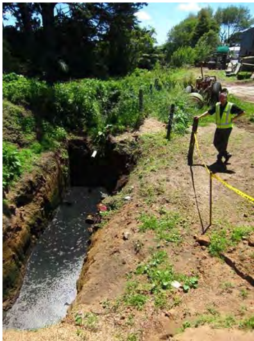
Photo 2 The new third settling pond, 2 December 2014
