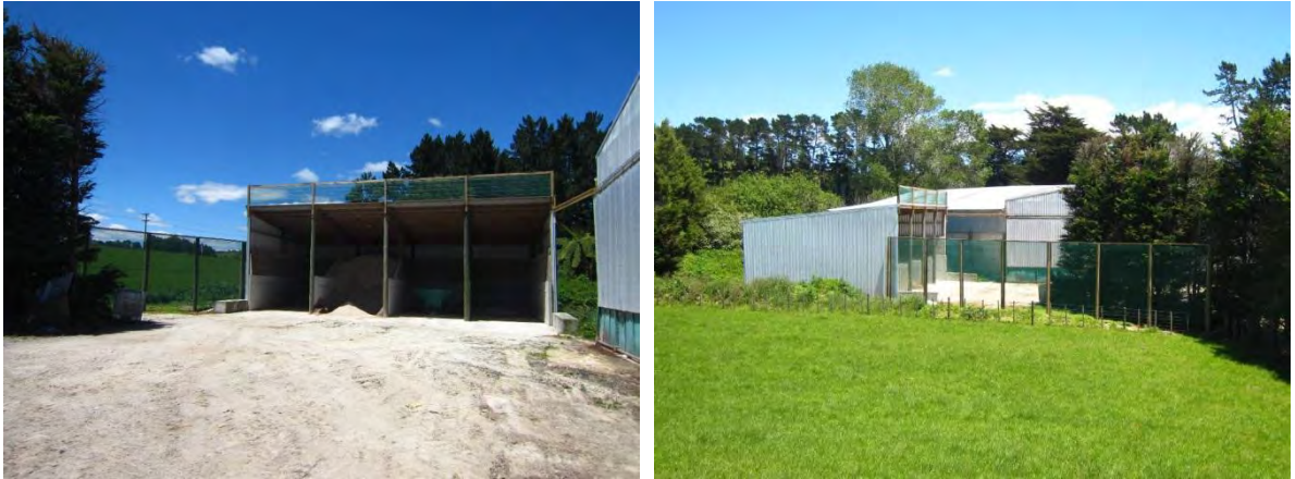
Photo 3 Extension of odour control system, and wind break, 2 December 2014
