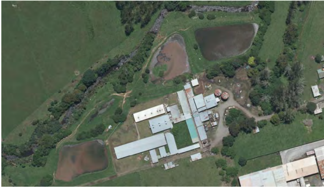
Figure 1 Aerial photograph of the piggery and wastewater treatment ponds
