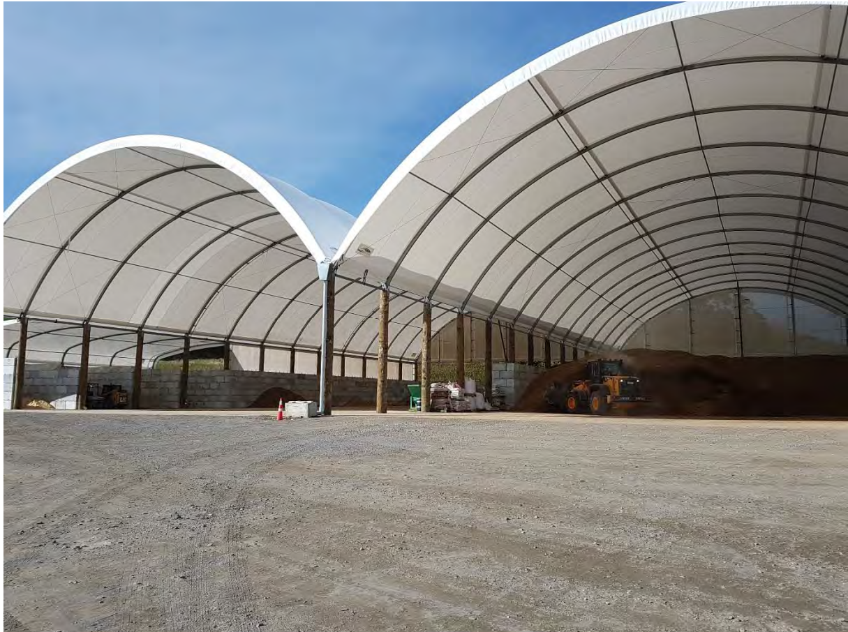
Figure 3 Osflo new site facility storage area 1319 Mountain Road
