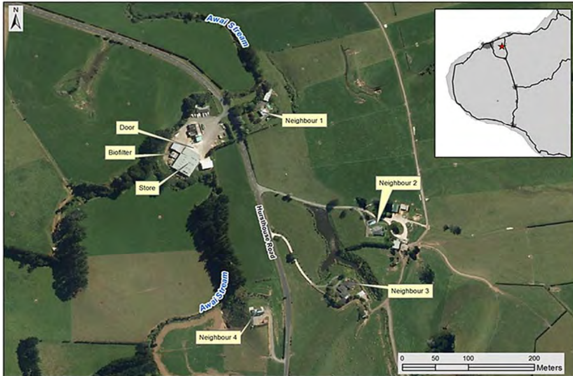
Figure 1 Osflo Fertiliser Ltd (former) site on the Hursthouse Road
