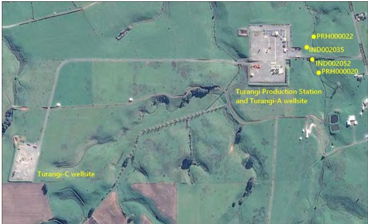
Figure 1 Turangi Production Station and associated sampling sites
