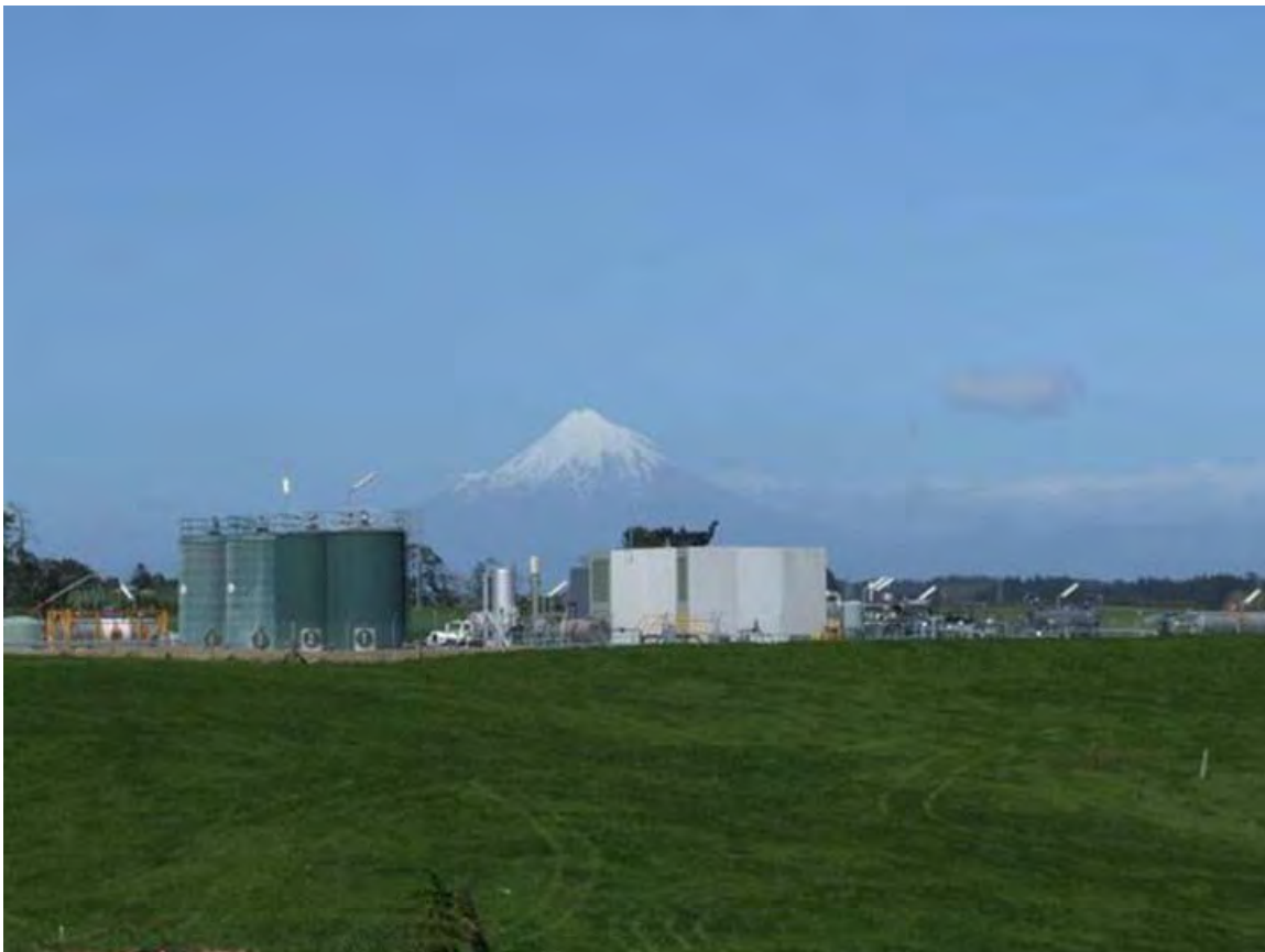
Photo 1 Turangi Production Station
