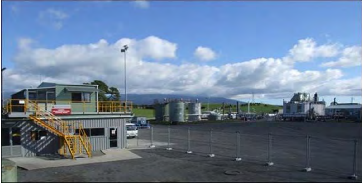
Photo 1 Kaimiro Production Station
