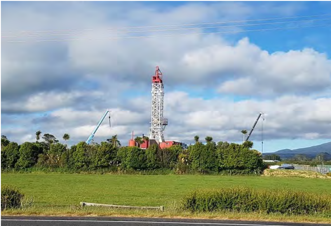
Photo 2 Radnor Production Station
