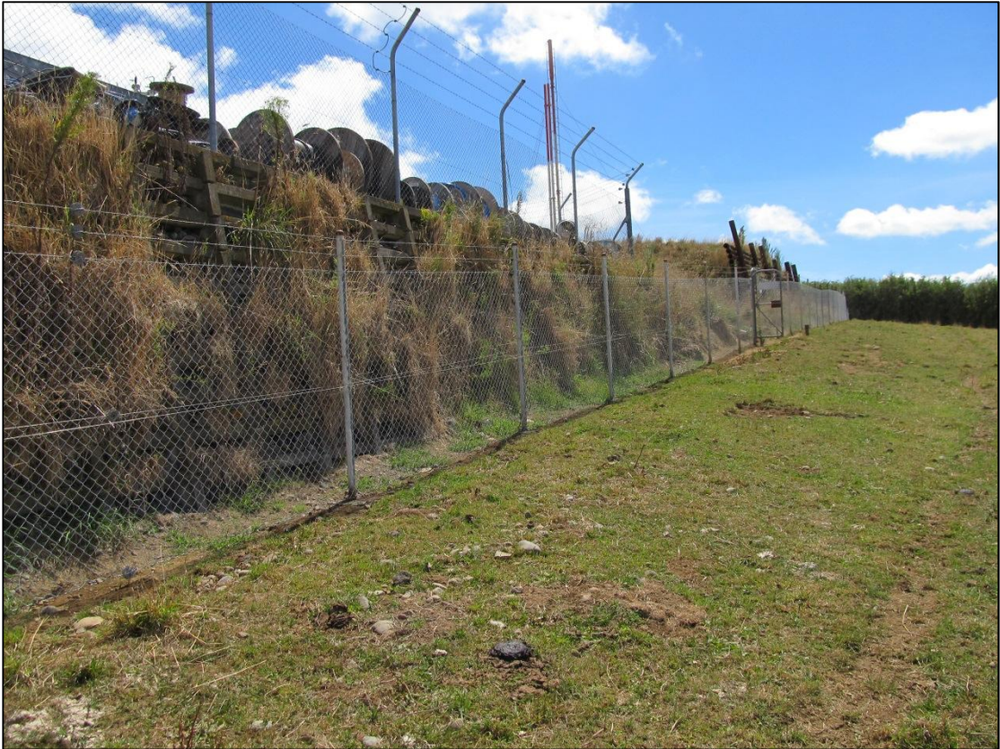
Photo 1 Boundary of wellsite KA-19/20 where the discharge from site occurred
