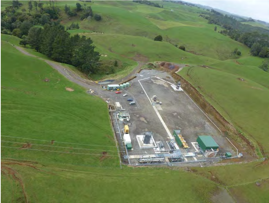
Photo 2 Kowhai-A Production Station
