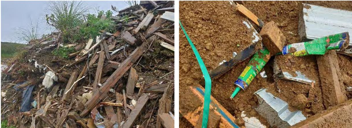
Photo 11 Unauthorised material in cleanfill including tin, wire, painted timber and Selley's packaging, June 2019
