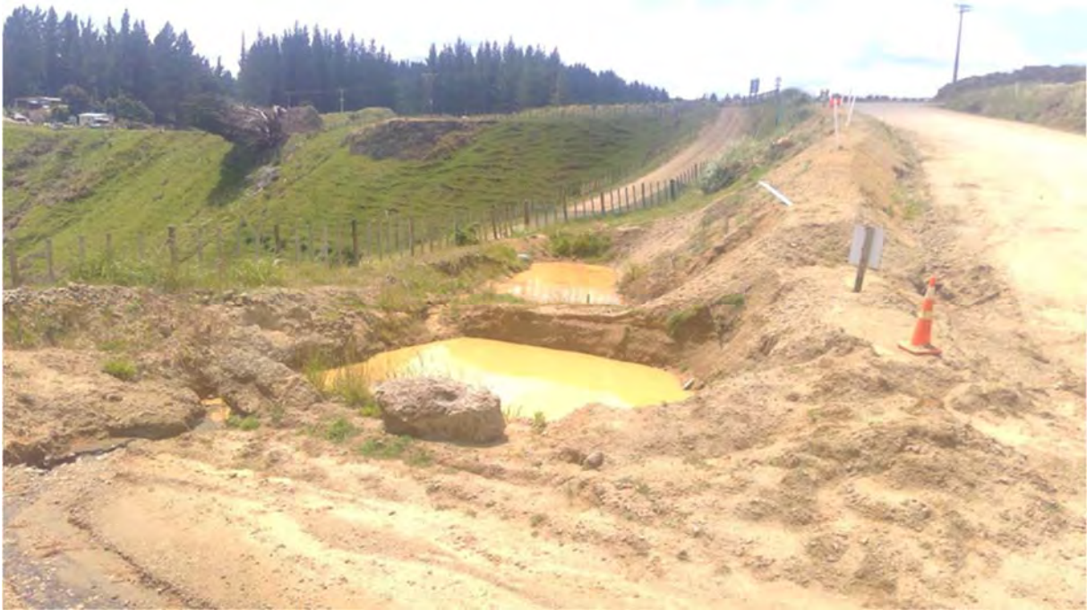
Photo 12 Two small treatment ponds on the east side of the site. Insufficient for the entirety of the site
