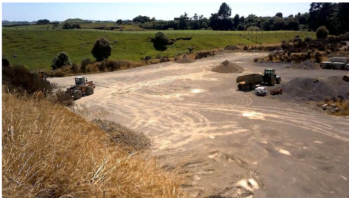
Photo 18 Taunt Contracting Ltd Bird Road quarry site 6 December 2017
