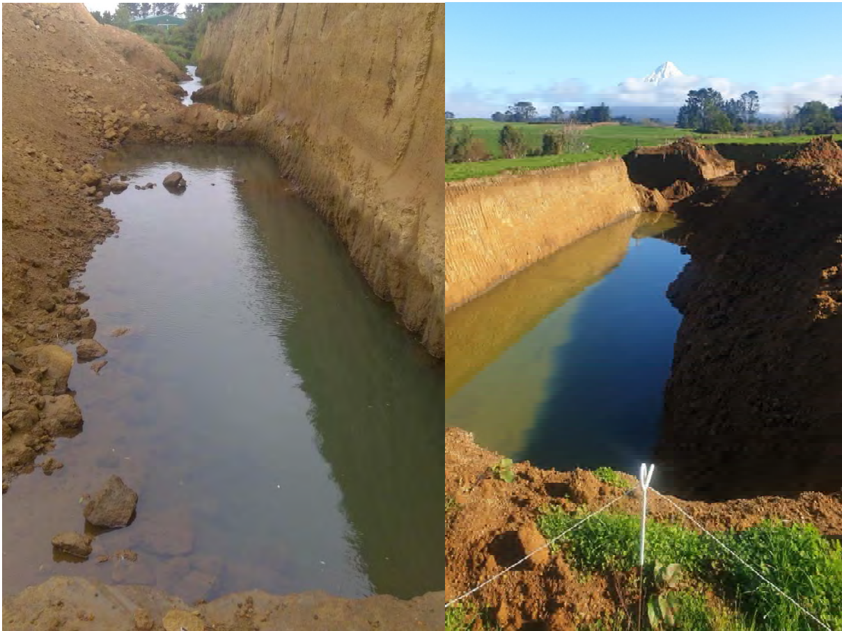
Photo 6 Hey Trust Quarry settling pond and drain as of December 2019 (left) discharging towards the Kahouri Stream. Settling pond drain as of May 2020 discharging to the unnamed tributary (right) rather than the Kahouri stream
