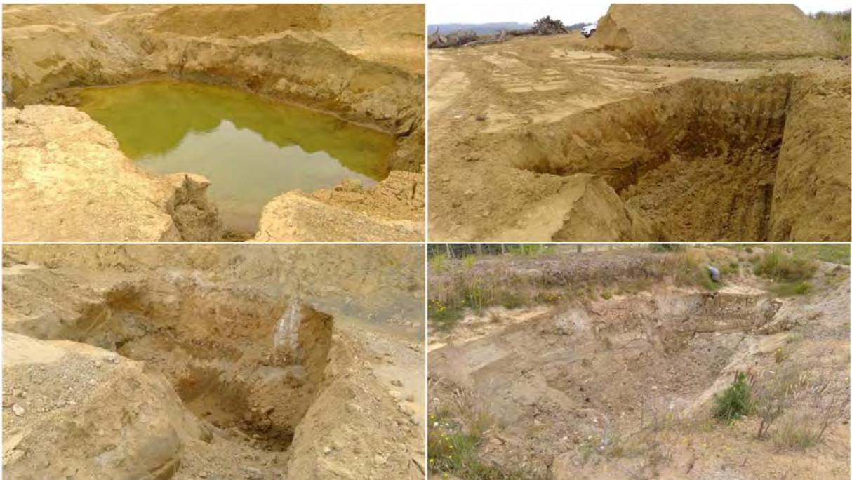
Photo 13 Settlement ponds added after abatement notice providing 745 m 3 for treatment of stormwater
