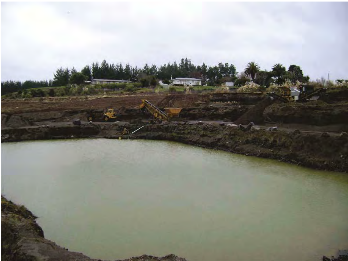
Figure 3 AA Contracting Ltd main settling pond
