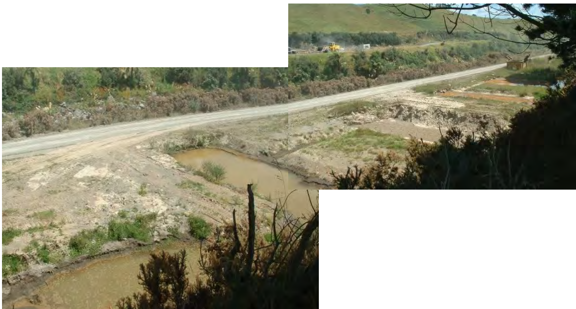
Figure 14 Sediment ponds at Whitaker Civil Engineering Quarry
