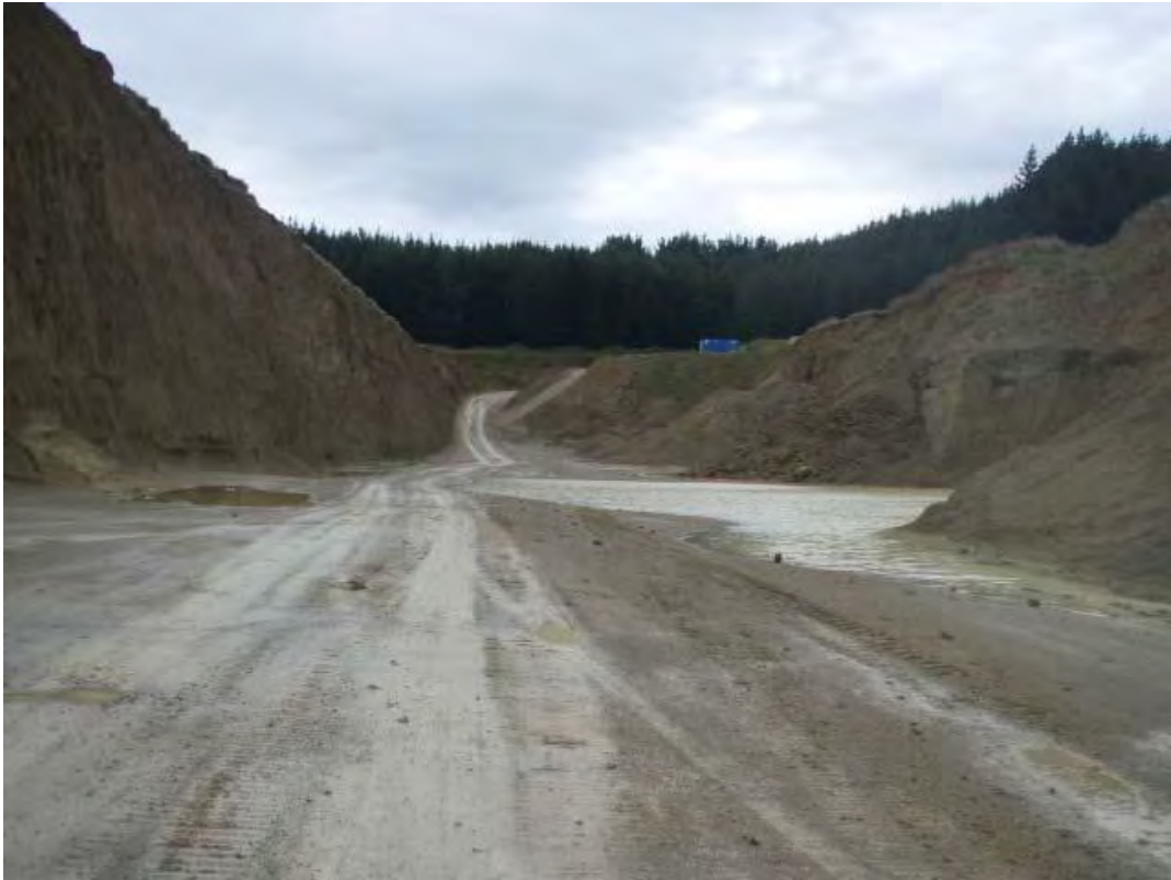
Photo 1 Stormwater collection area at base of quarry pit from which stormwater drains via seepage to ground
