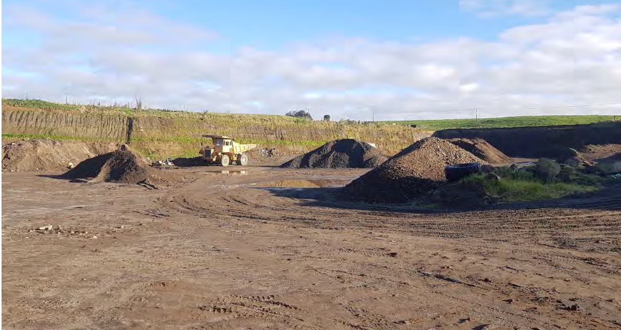
Photo 1 AA Contracting Ltd Quarry pit July 2018
