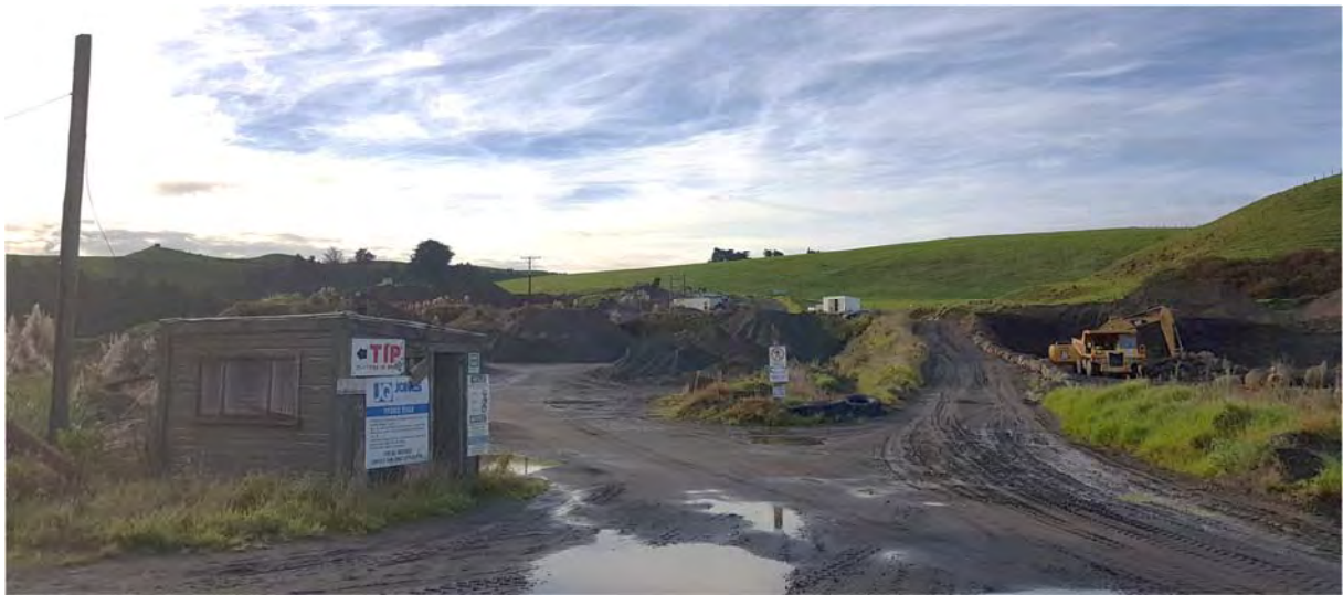
Photo 8 Hydro Road quarry and cleanfill from site entrance
