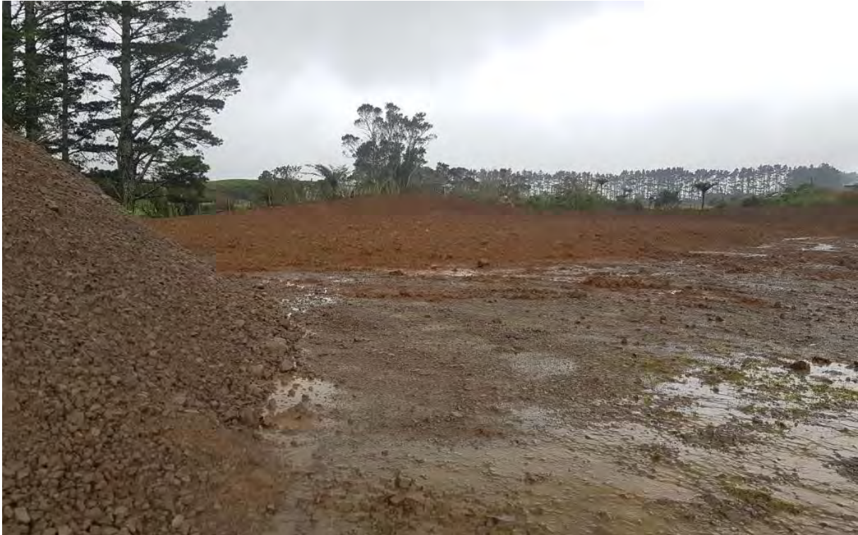
Photo 5 Reinstated Gibson Family Trust Newall Road site
