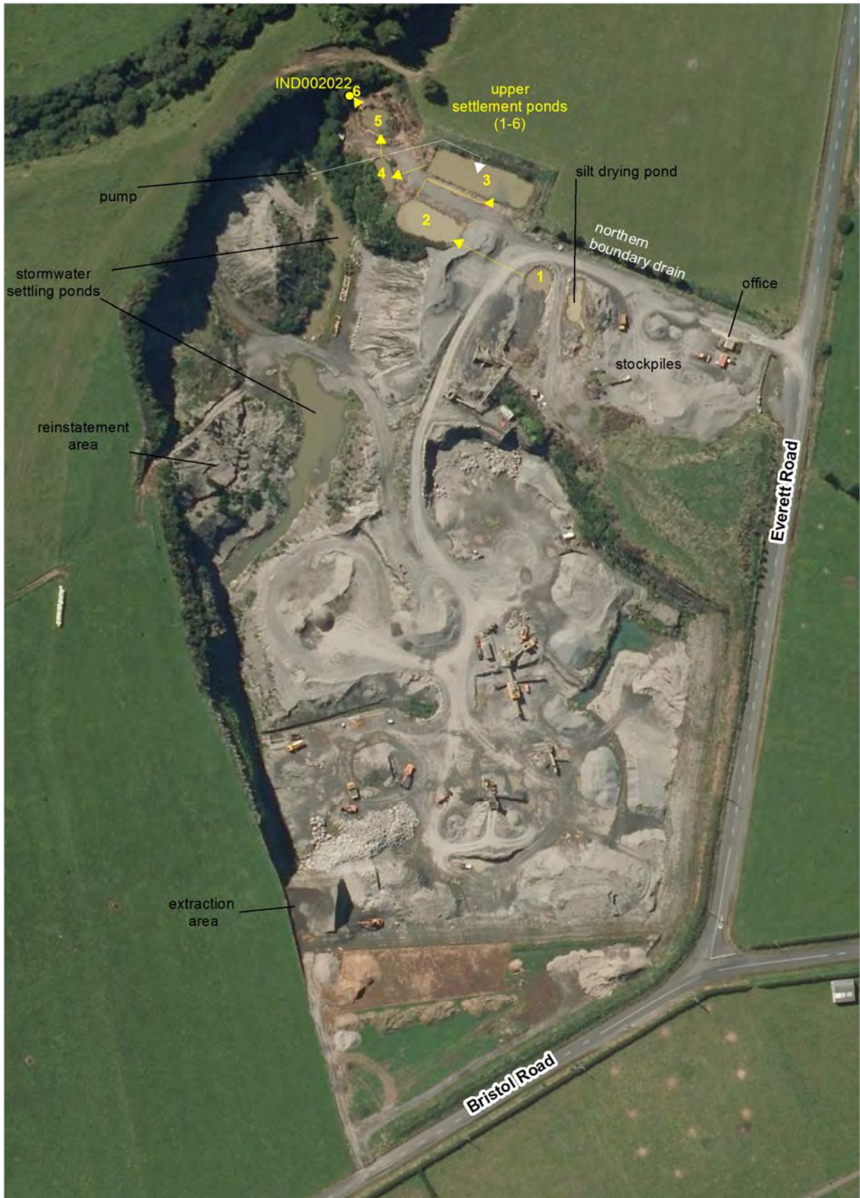
Figure 1 Quarry operations, wastewater treatment system, Everett Road Quarry
