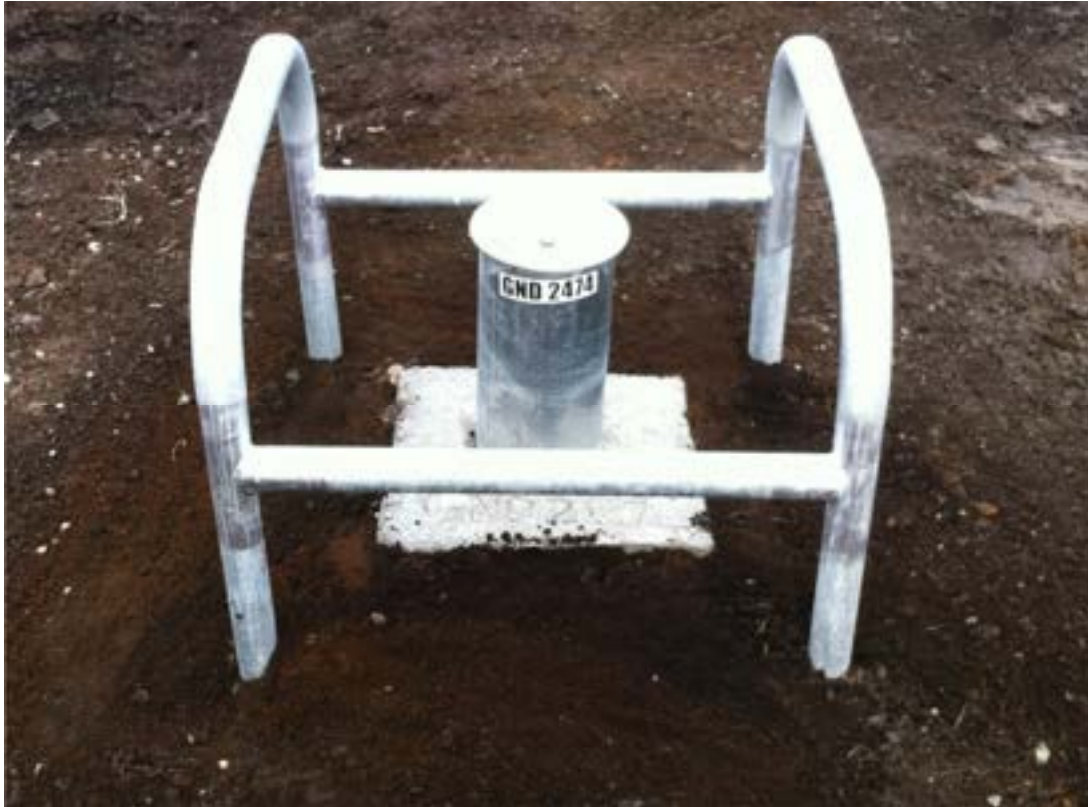
Headworks of a groundwater bore.
