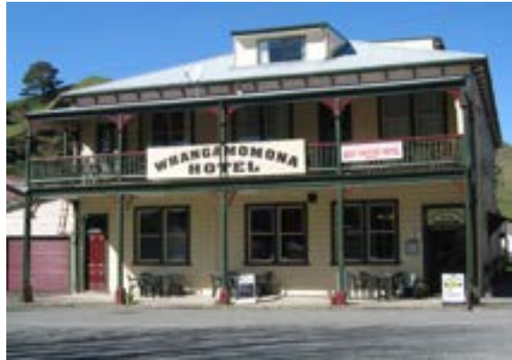
The Whangamōmona Hotel, the second hotel on the site, was built in 1911.
