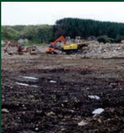
Removal of above-ground structures.
