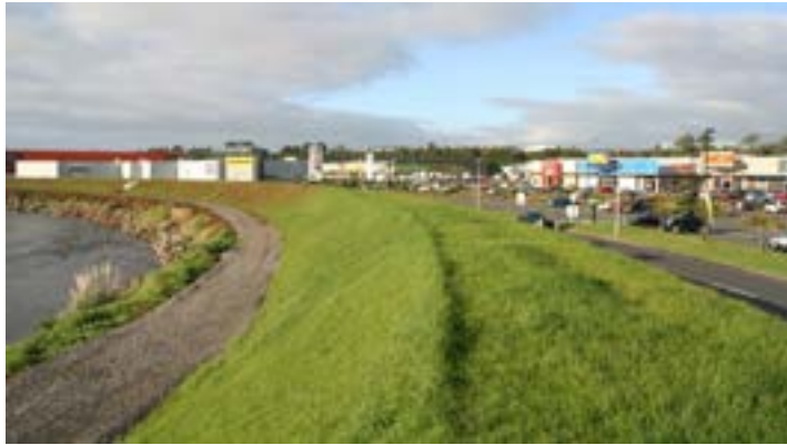
Stopbanks along the Waiwhakaiho River protect the shopping centre.
