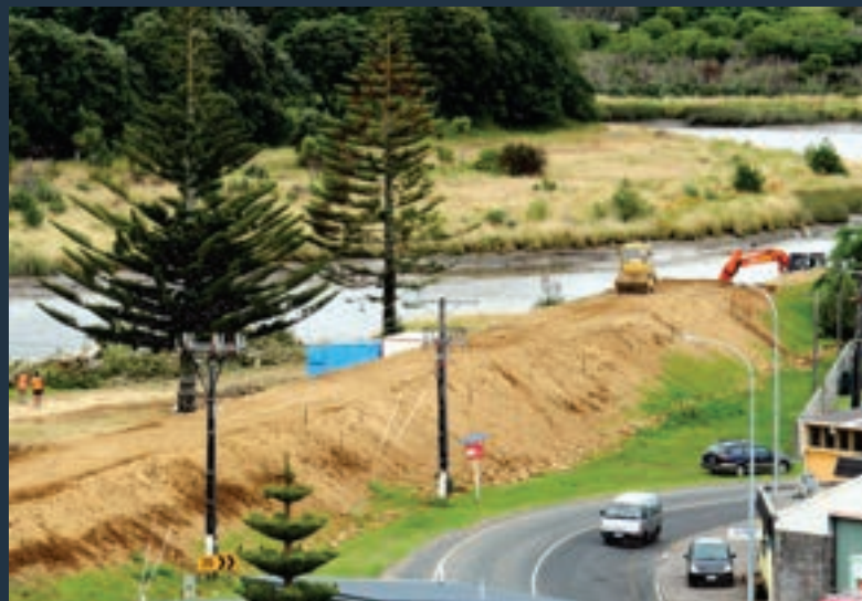
Earthen stopbanks being raised north of the Town Bridge.
