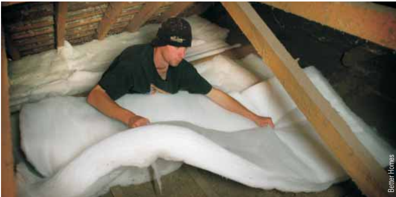
Harley Meston of Better Homes installing ceiling insulation.
