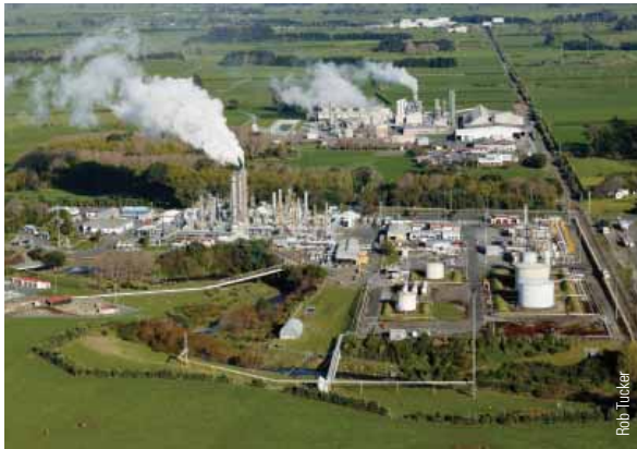
Vector Kāpuni gas treatment plant (foreground) and Ballance ammonia-urea plant, Kāpuni.
