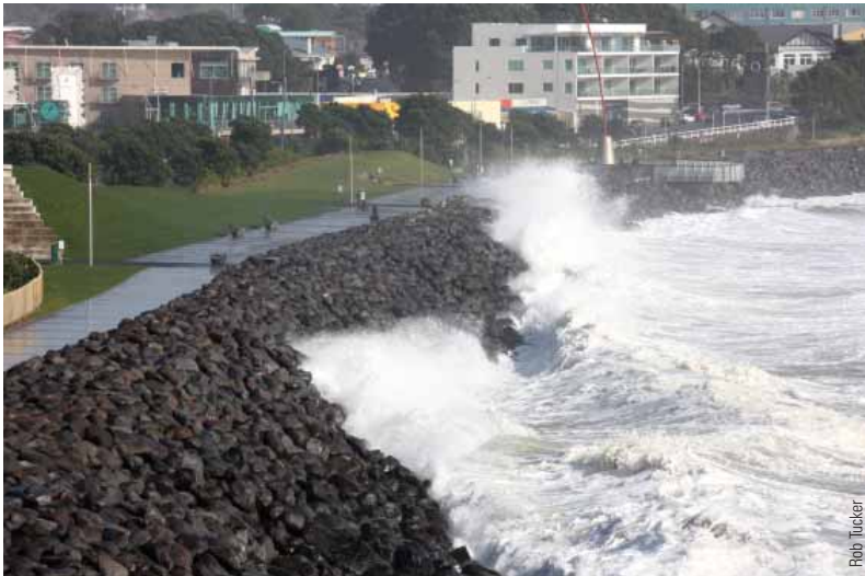
Coastal walkway and sea wall, New Plymouth.
