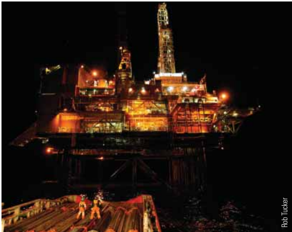
Maui A production platform and supply vessel, offshore from Opunake.
