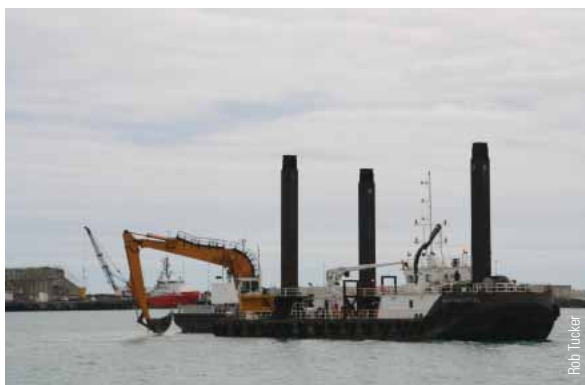
Dredging in Port Taranaki.
