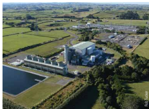
Stratford combined cycle power station.
