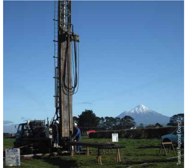
Drilling a water bore, Eltham.
