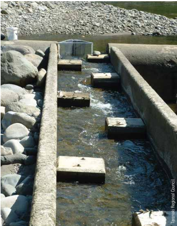
Fish pass on the Waiwhakaiho weir.
