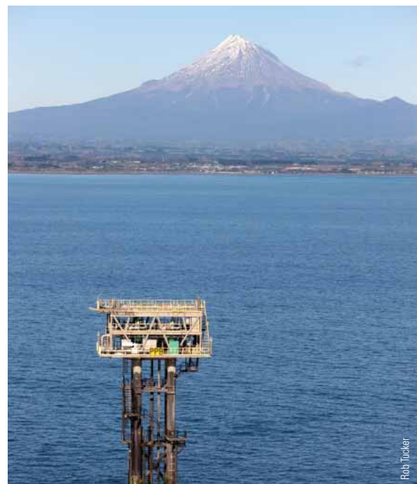
Pohokura offshore well-head platform.
