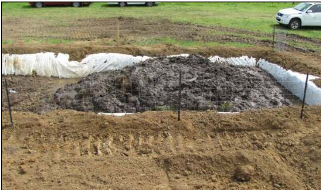
Photograph 7 – Contaminated soil storage pit – 19 October 2010
