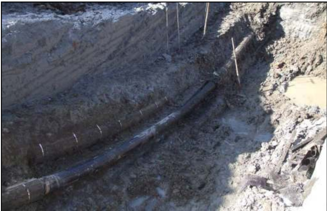
Photograph 11 – Excavation of the pipeline – 27 October 2010
