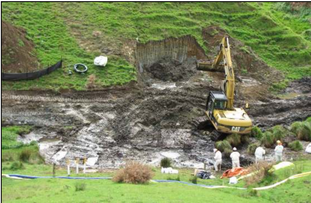
Photograph 6 – Removing the contaminated soil from the pipeline route– 18 October 2010
