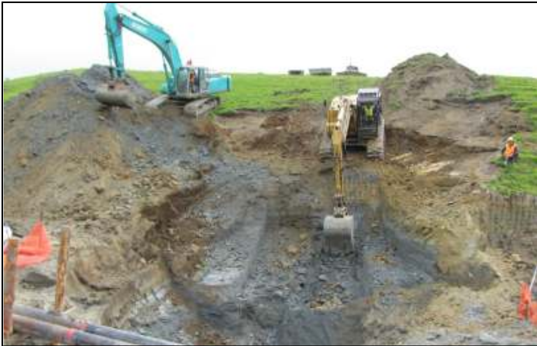
Photograph 12 – Diggers removing the soil – 2 November 2010
