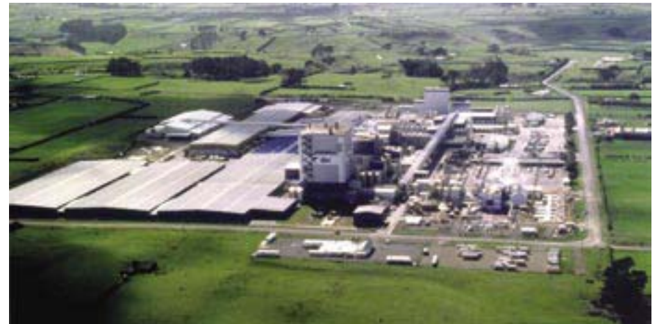
Photo 5: Fonterra Group Cooperative Ltd's Whareroa dairy processing site near Hawera
