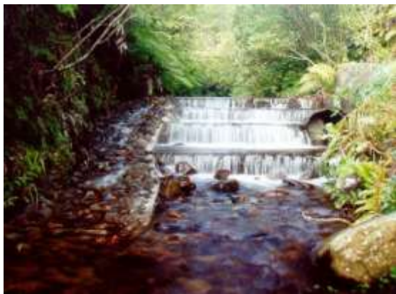
Fish passes allow fish to migrate past the structure like this one on the Wairau Stream
