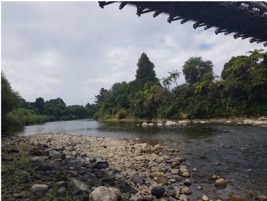
Figure 3: Slow run habitat in the Waitara River downstream of the Bertrand Road Bridge at a flow of 5.1 m 3 /s.
