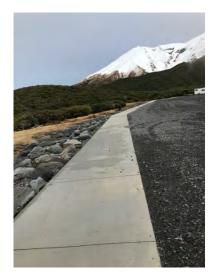
construction of a concrete footpath around the perimeter of the carpark, placing rocks to control surface water run-off and sealing of the carpark surface. Unfortunately, the cold weather beat us, resulting in the carpark not being sealed. This will be undertaken later this year, when weather conditions are more suitable for sealing.
