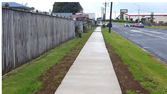
Footpath renewal work completed in Tasman Street, Opunake.
