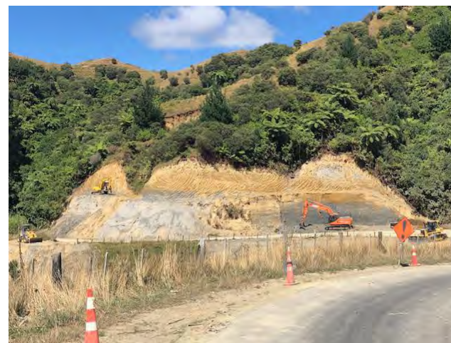
Mangaotuku Road Realignment
