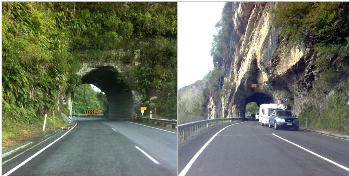
The two tunnels on the route – on Mount Messenger (left) and the Awakino Gorge (right), April 2014
