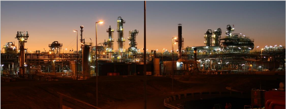
Taranaki's oil and gas industry at work - Kupe Production Station at dawn
