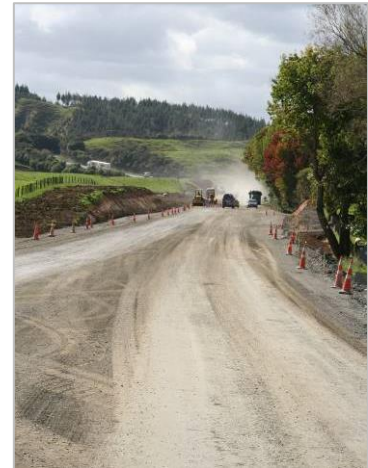
Construction of Awakino northbound passing lane
