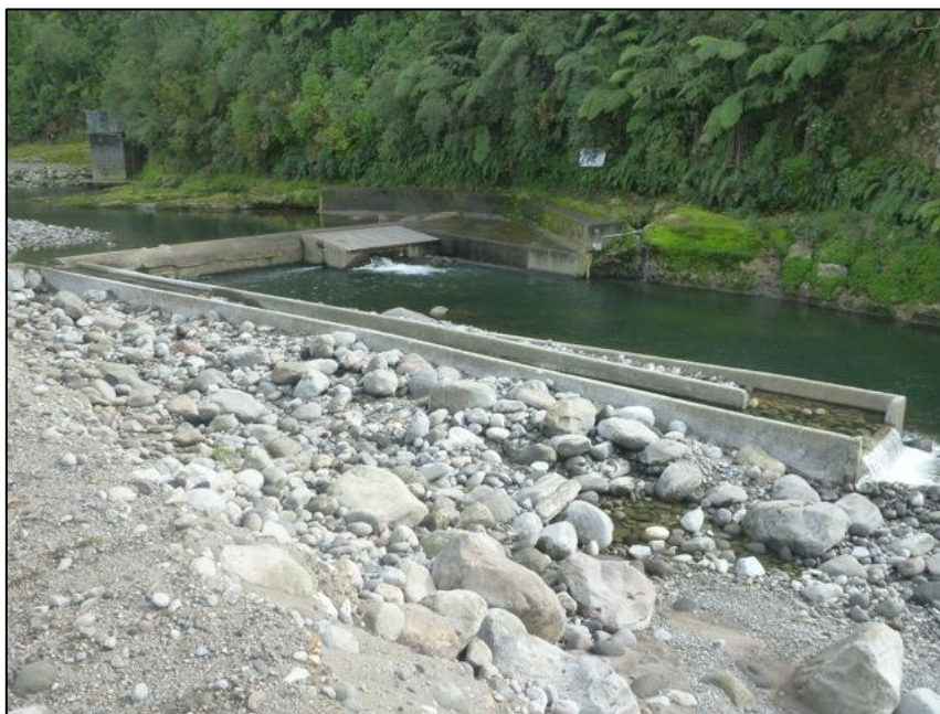
Figure 10. Mangorei HEPS diversion weir with fish pass in the foreground (blocked by boulders due to flooding).
