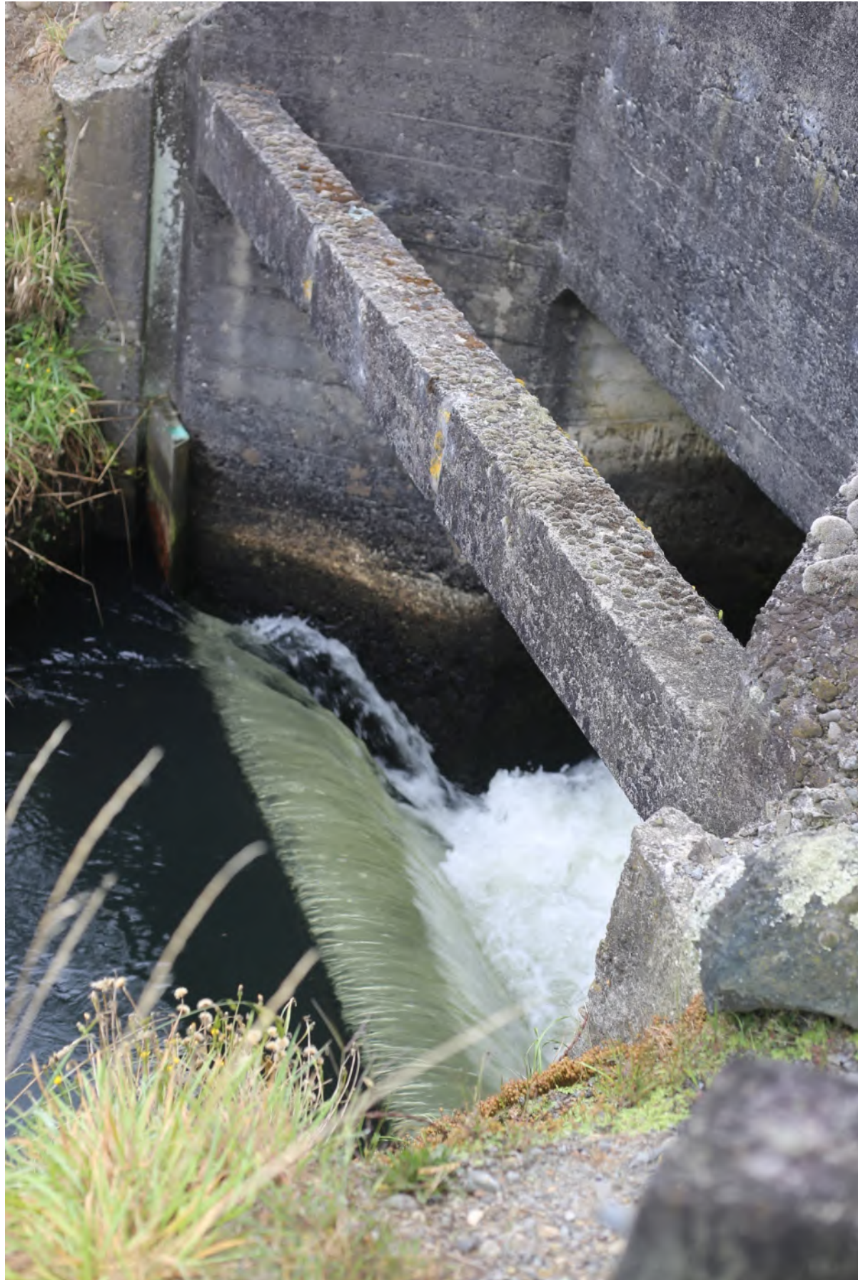
Tariki Road Weir
