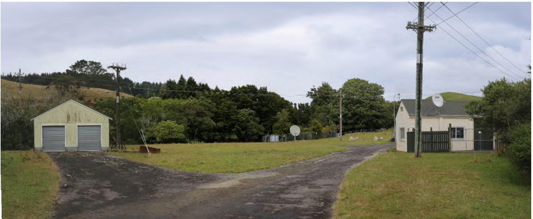
Power Station and Surrounds
