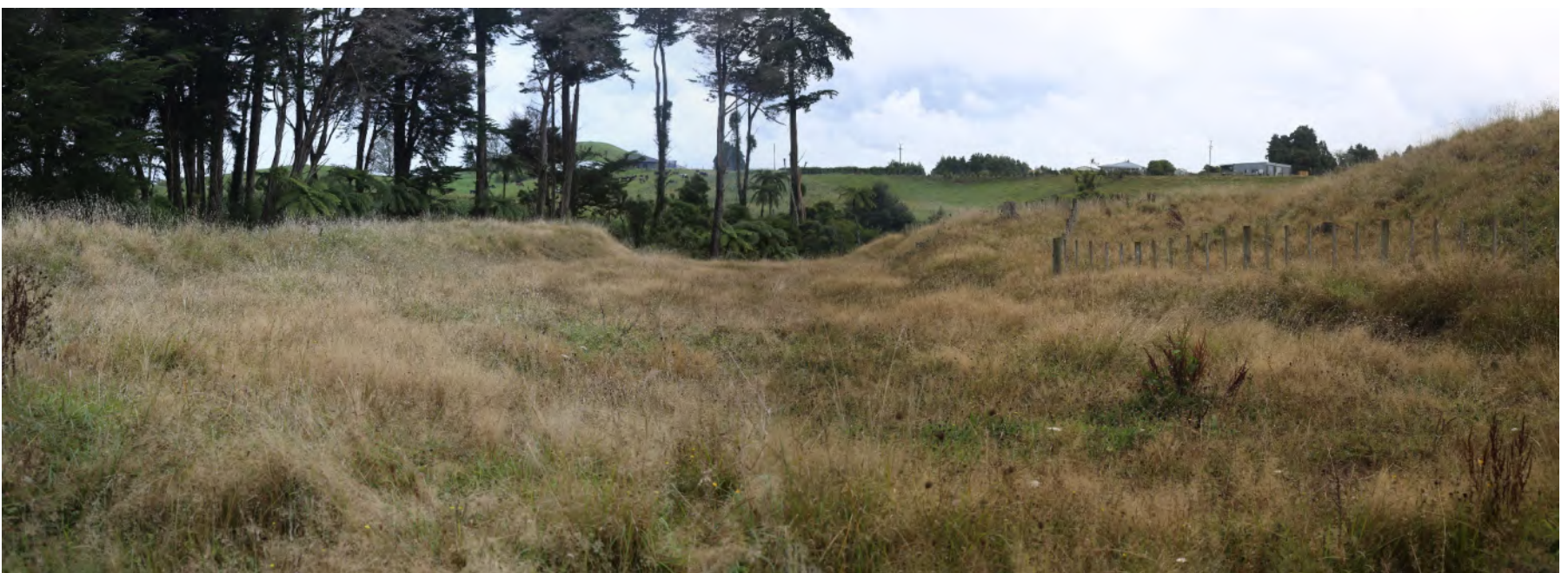
Mako Stream Emergency Spillway
