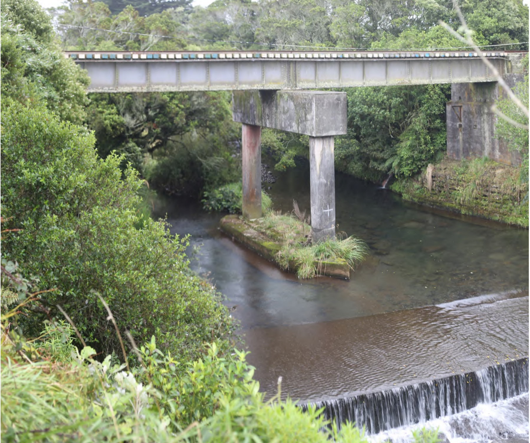
Weir at SH3 / Rail Crossing
