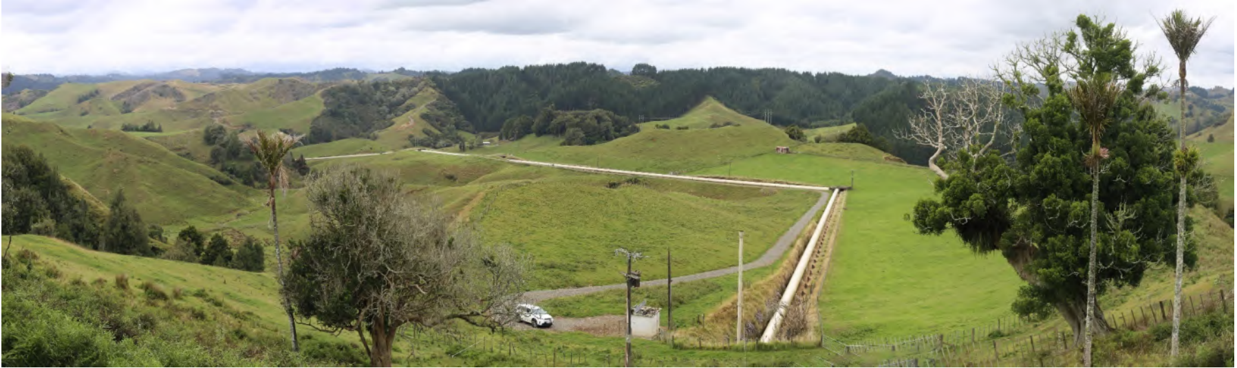
Penstock Below Surge Chamber
