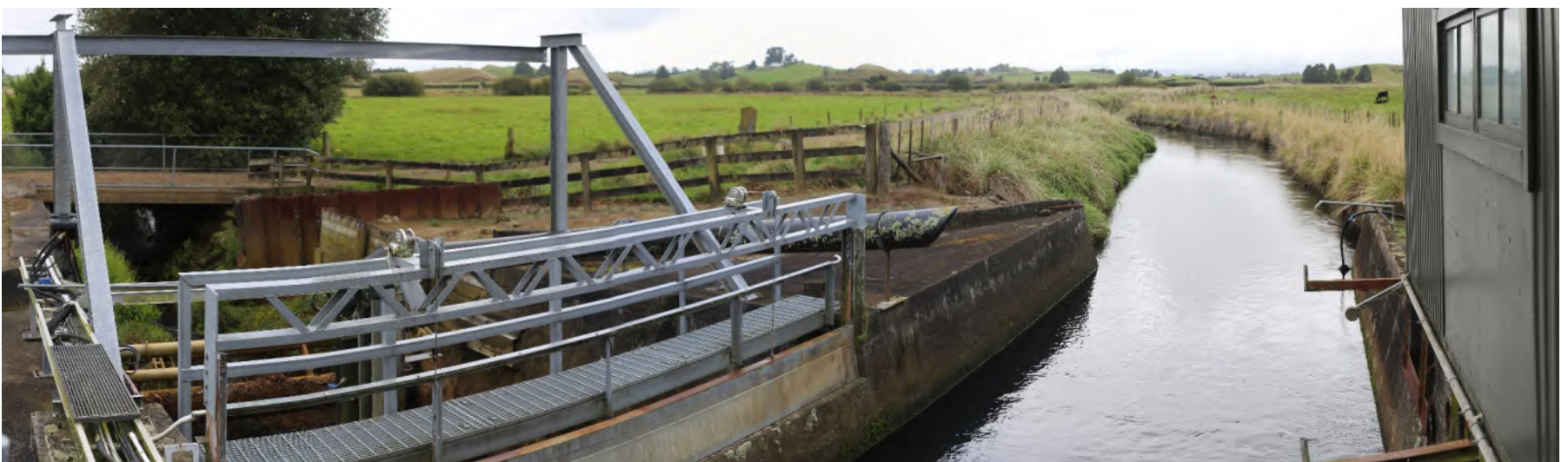
Mangaotea Stream Aqueduct
