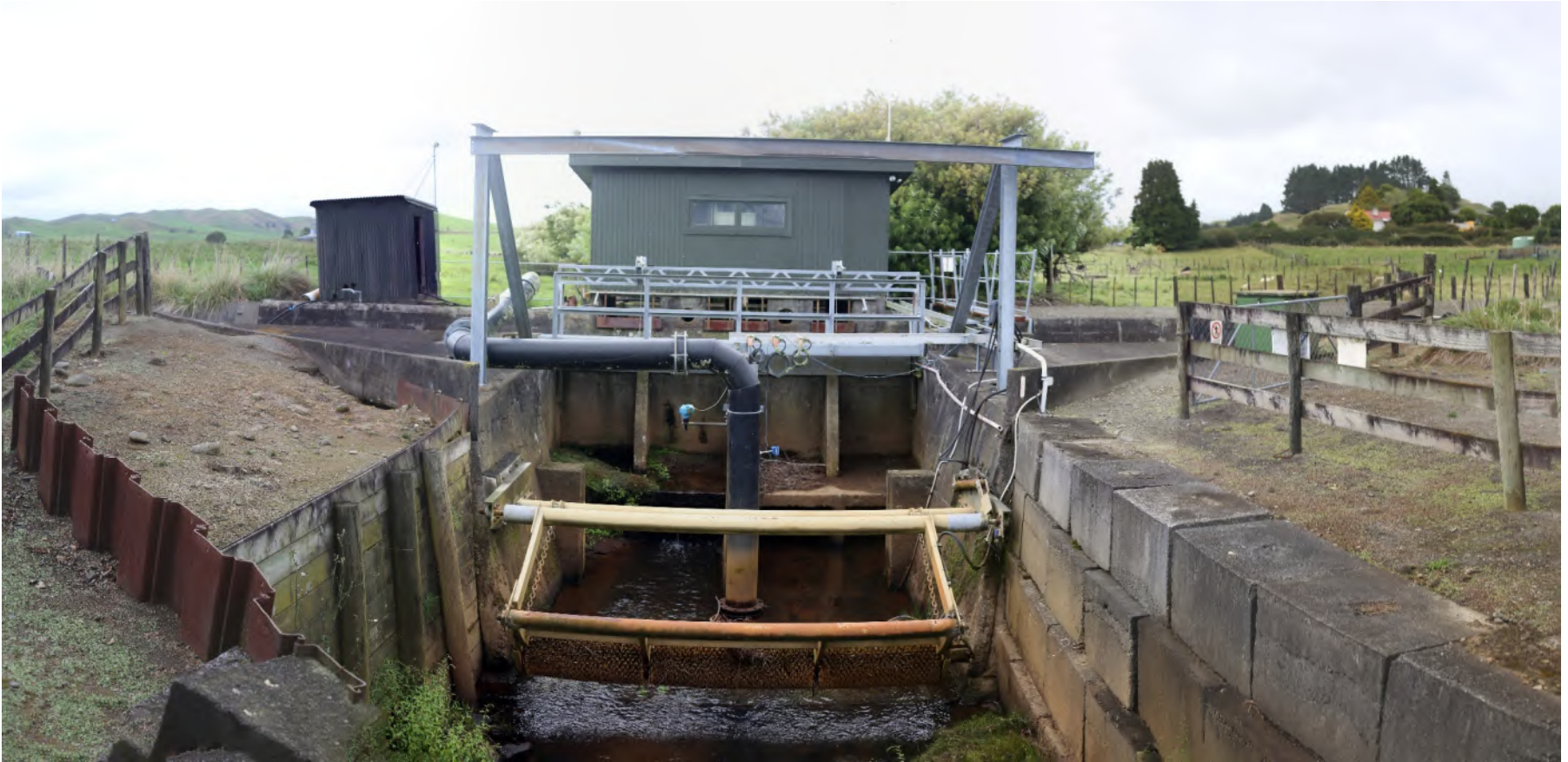
Mangaotea Stream Aqueduct
