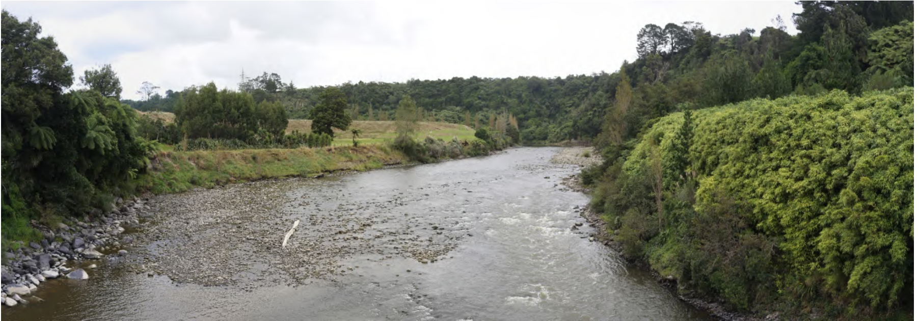
Bertrand Road Bridge (Upstream)
