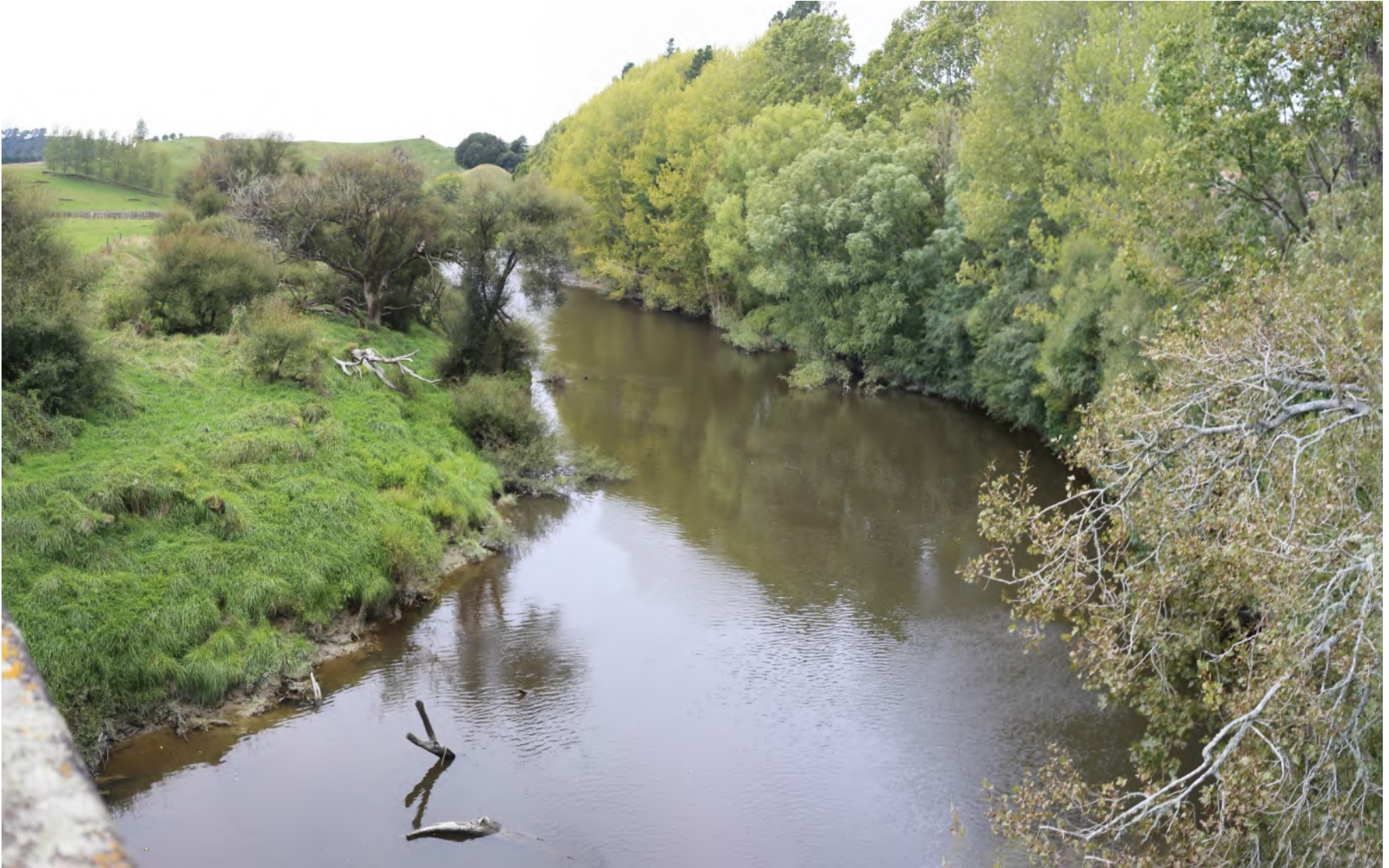
Tarata Road Bridge (Upstream)
