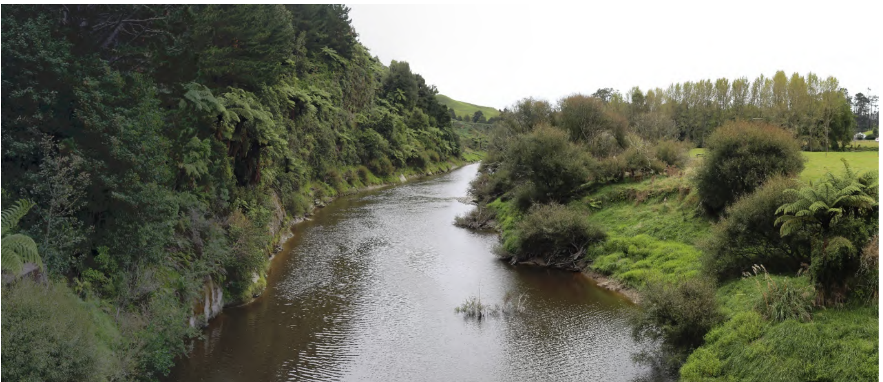
Tarata Road Bridge (Downstream)
