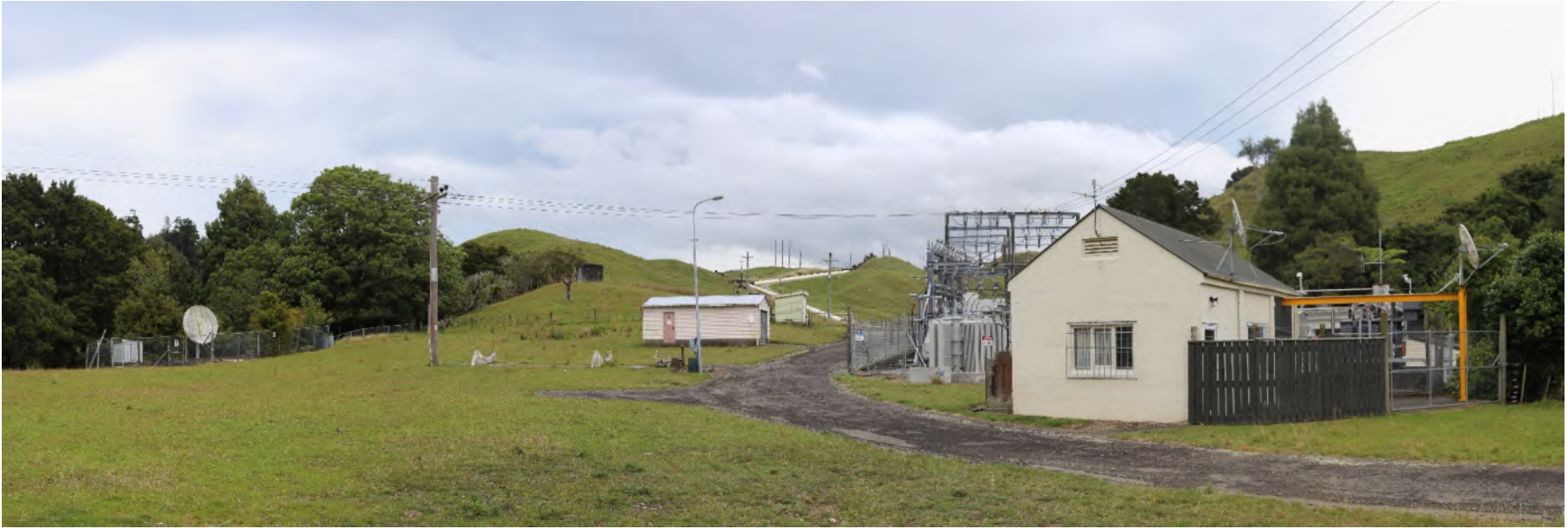
Power Station and Surrounds
