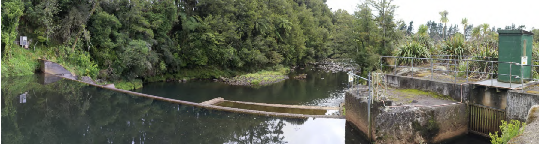
Weir and Intake Structure
