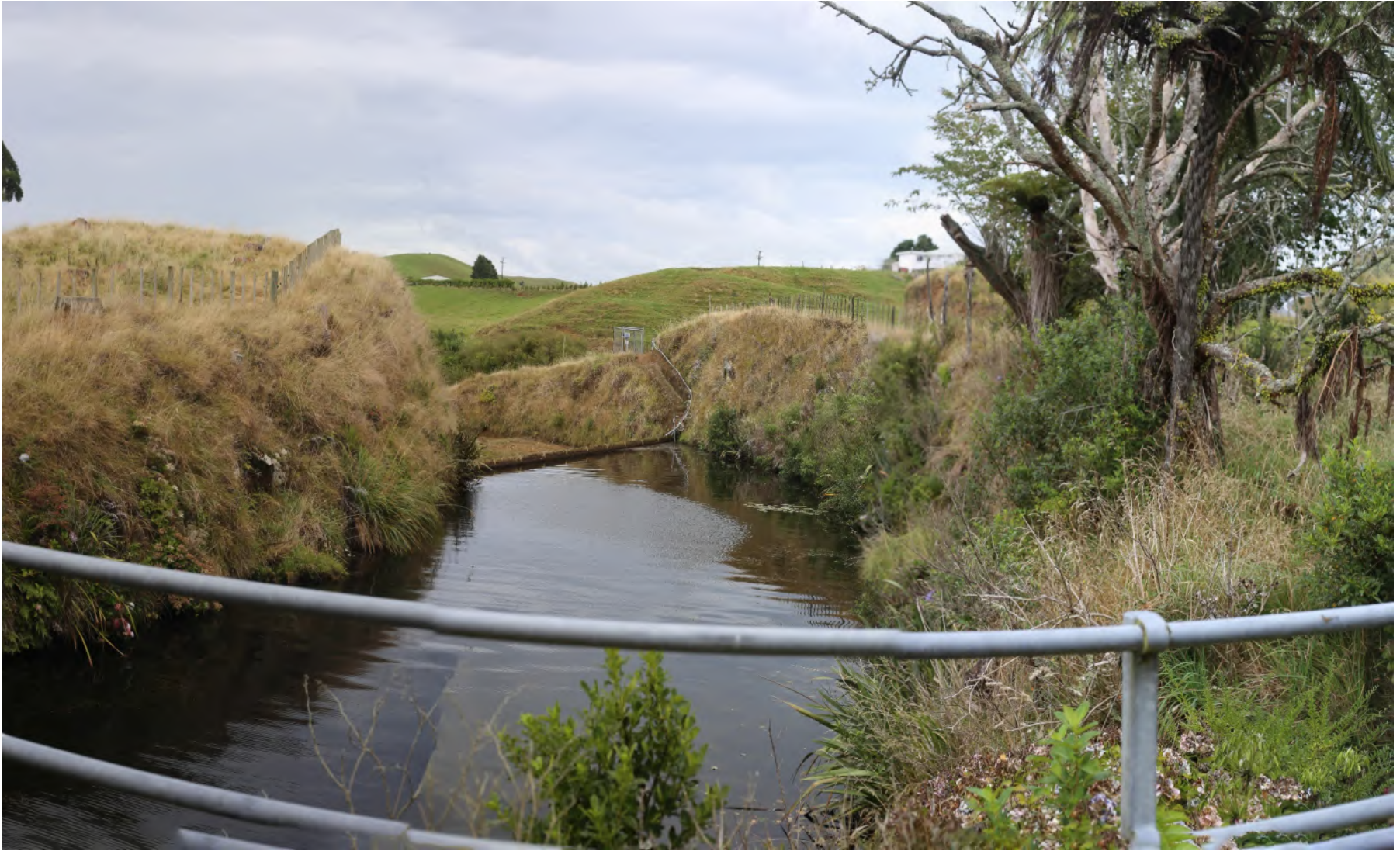
Mako Stream Service Spillway
