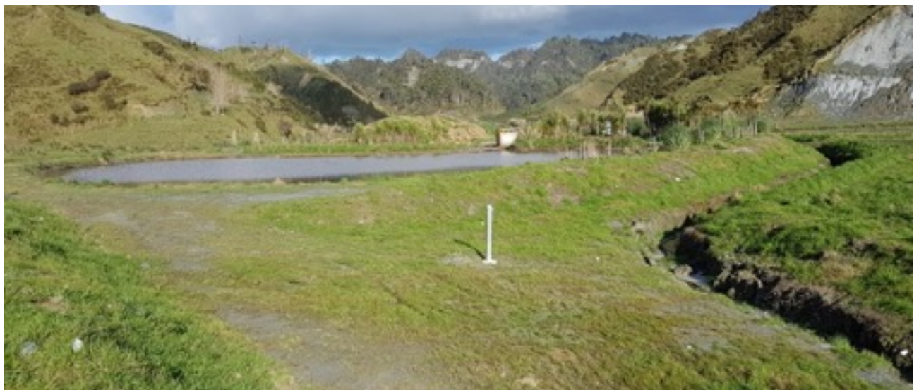
Figure 13. Exclusion Drain (right) diverts clean water around the 'duck pond'
